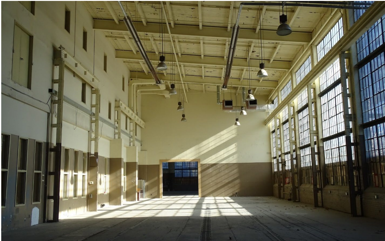
Figure 32: Interior photograph of 185 Eastern Avenue looking east, showing the south half of the building and large industrial window units along Palace Street. The interior demising wall that divides the building along the ridgeline of the roof is on the left of the photograph and the 1947 addition is visible through the large opening in the interior partition that divides the main space of the 1929 building. (SBA Ltd., 2021)
