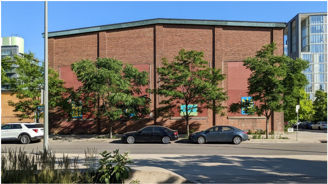
Figure 36: North elevation of 153 Eastern Avenue. (Heritage Planning, 2022)
