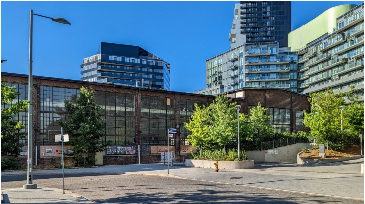
Figure 25: Partial south elevation of 185 Eastern Avenue showing the eastern addition. (Heritage Planning, 2022)
