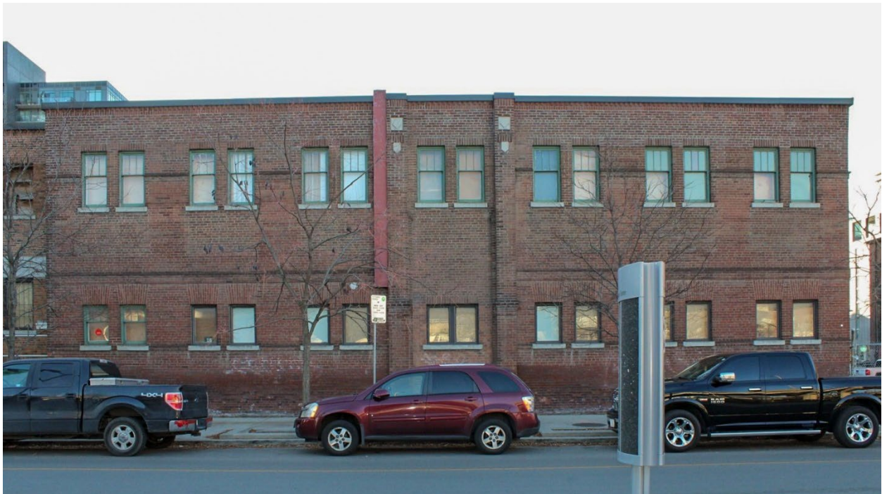
Figure 16: The north elevation of 169 Eastern Avenue, prior to demolition in 2021. (SBA Ltd., 2021)
