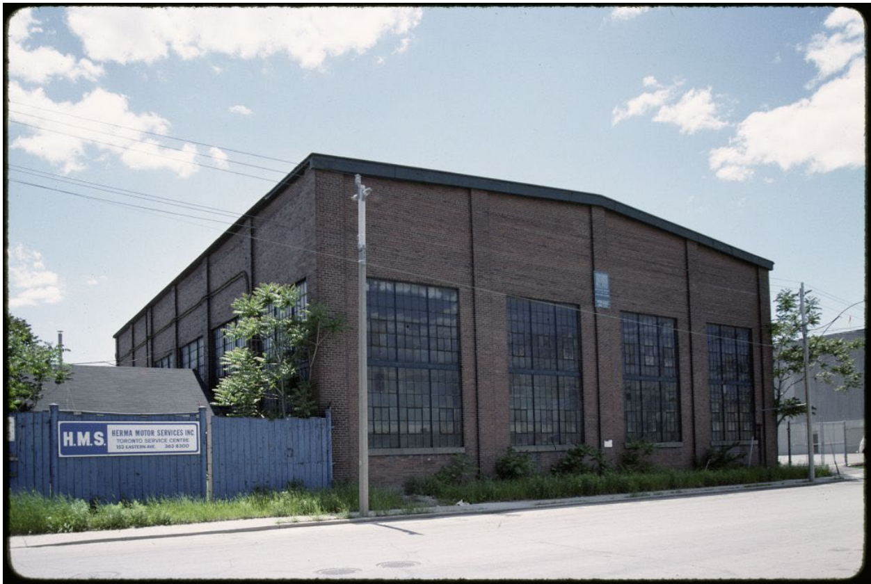
City of Toronto Archives, Series 1465, File 667, Item 4 Figure 37: 1988-89 archival photograph showing the east and north elevations of 153 Eastern Avenue. (City of Toronto Archives)
