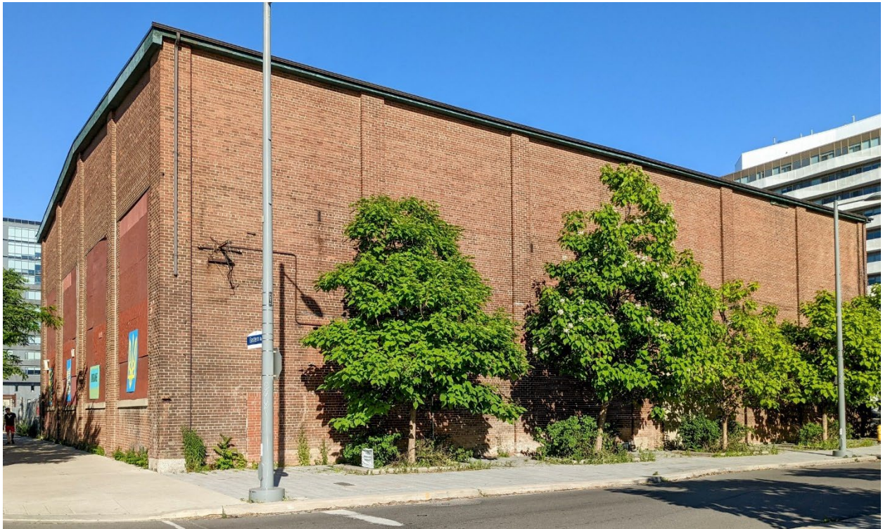
Figure 39: North elevation of 185 Eastern Avenue. (Heritage Planning, 2022)
