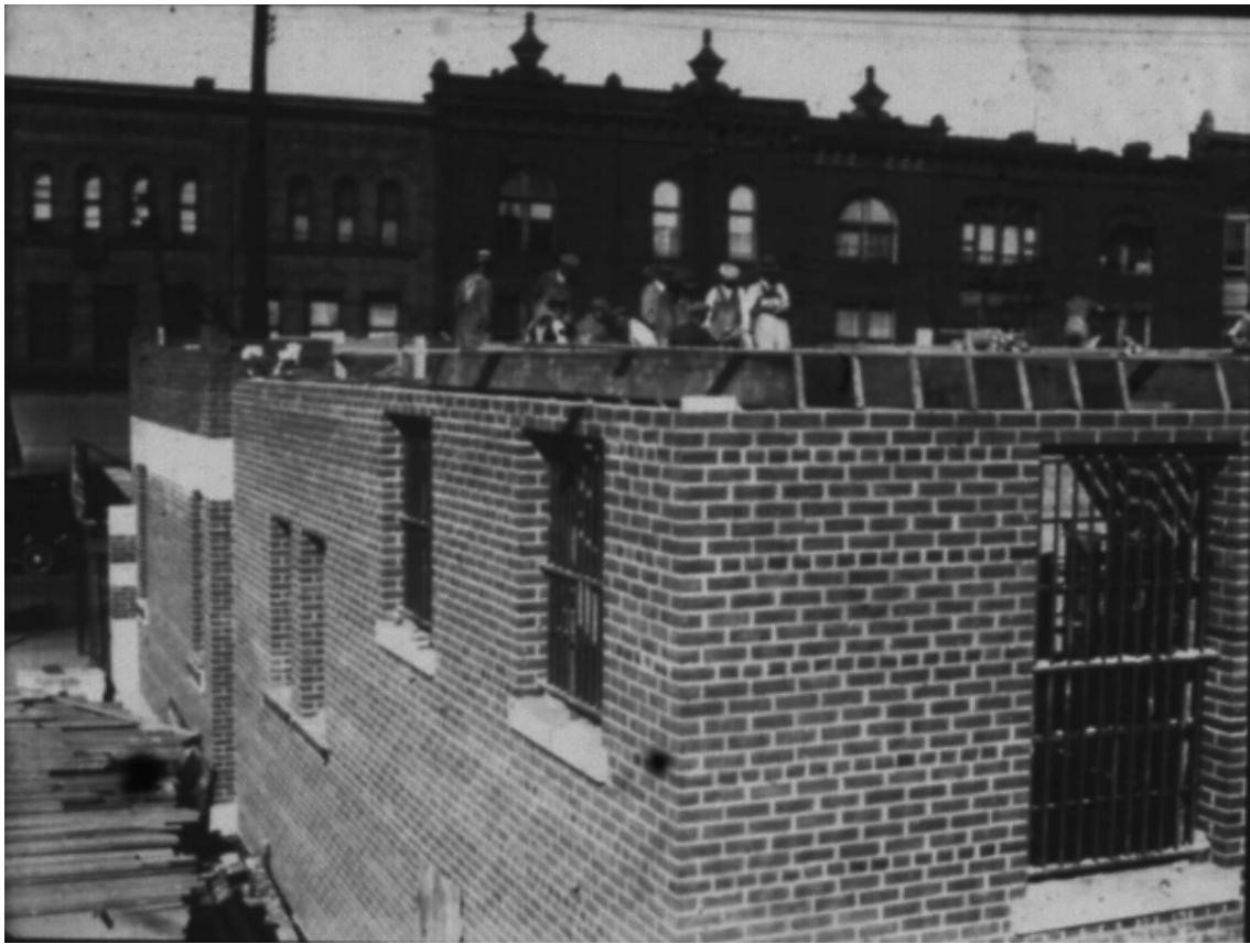
Figure 20: Archival photograph of 1313 Queen Street West under construction, showing the original window openings of the cell block (City of Toronto Archives; Fonds 1266, Item 25674).
