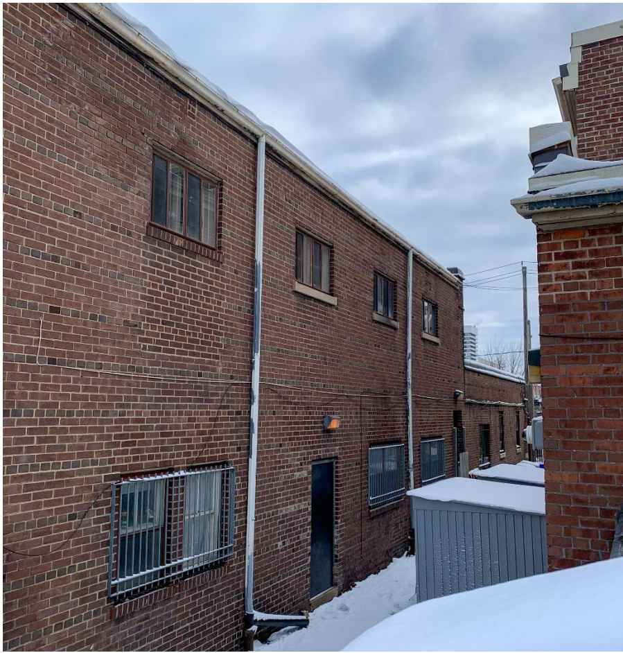
Figure 22: South (rear) elevation of the former stables, 1313 Queen Street West (Heritage Planning, 2023).
