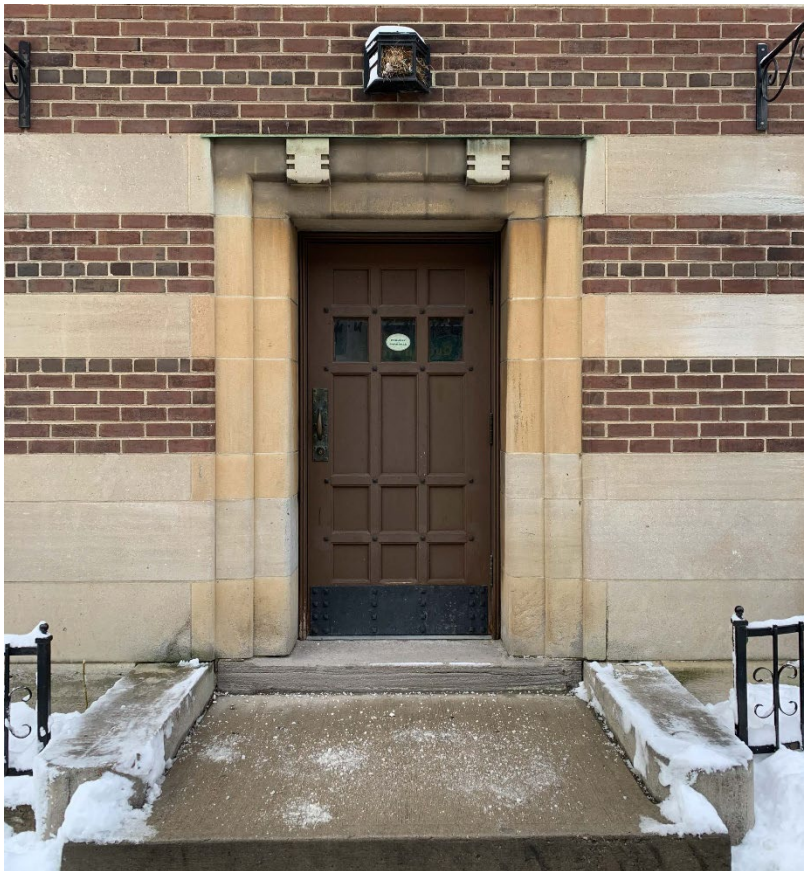
Figure 13: Secondary entrance on north elevation of 1313 Queen Street West (Heritage Planning, 2023).
