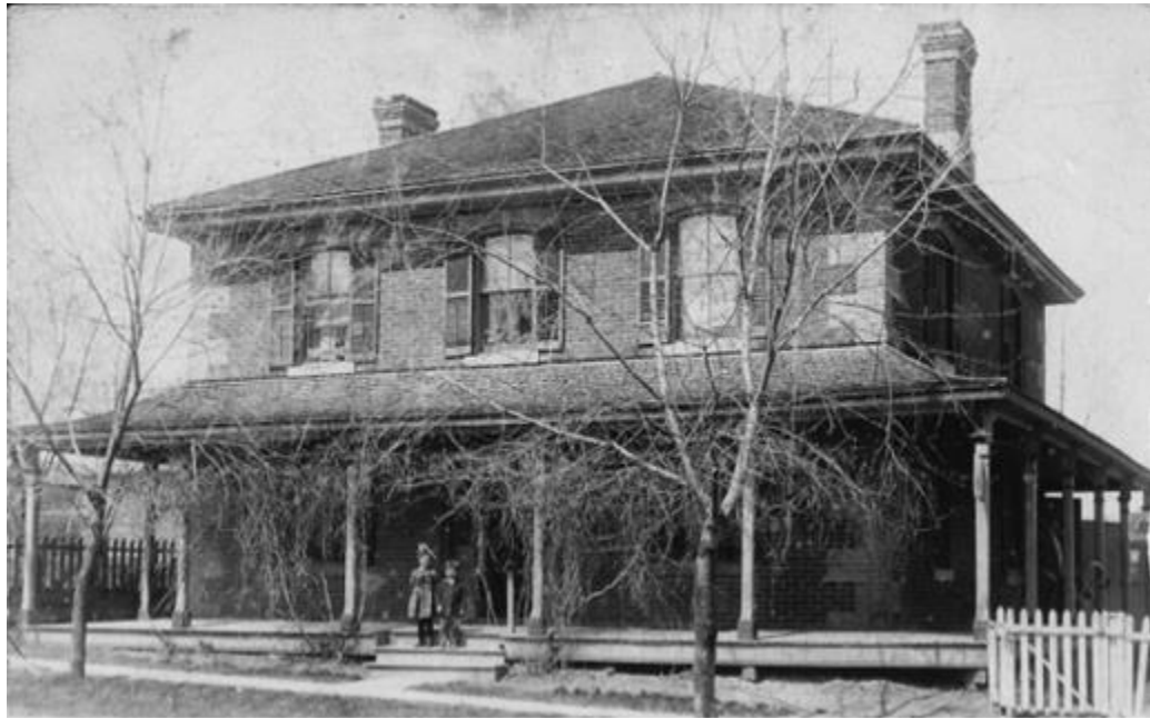
Figure 3: South (principal) façade of 4888 Dundas Street West, c. 1920 (Etobicoke Historical Society)
