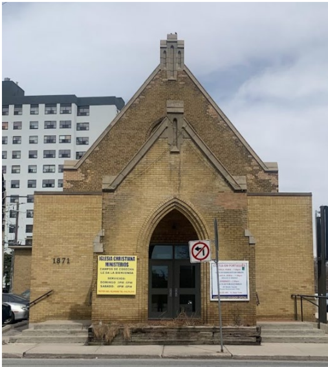
Images 32 and 33. Brick buttresses, stone coping and decorative stone gable treatments on south elevation and 1947 vestibule façade, at left; 1957 image of front vestibule showing original configuration including the rose transom, at right (Heritage Planning, 2023 and Weston Historical Society, respectively)
