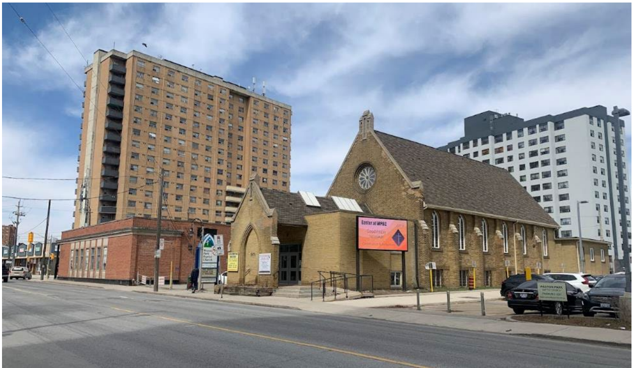
Image 51. View looking northeast across the site (Heritage Planning, 2023)
