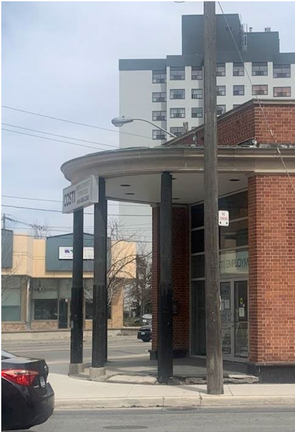
Image 47. The projecting curved front porch roof of the bank building supported on four precast granite (terrazzo) clad columns (Heritage planning, 2023)
