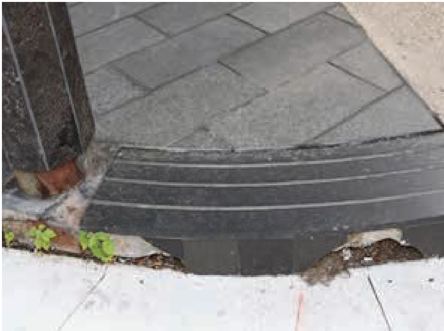
Image 48. Detail of the remaining granite treads and risers on the front porch (ERA, 2021)
