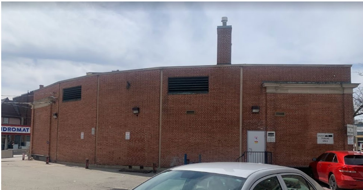
Image 46. Looking northeast at the rear elevation of the former bank building, noting the single-bay return of the limestone cornice supported by red brick pilasters (Heritage Planning, 2023)
