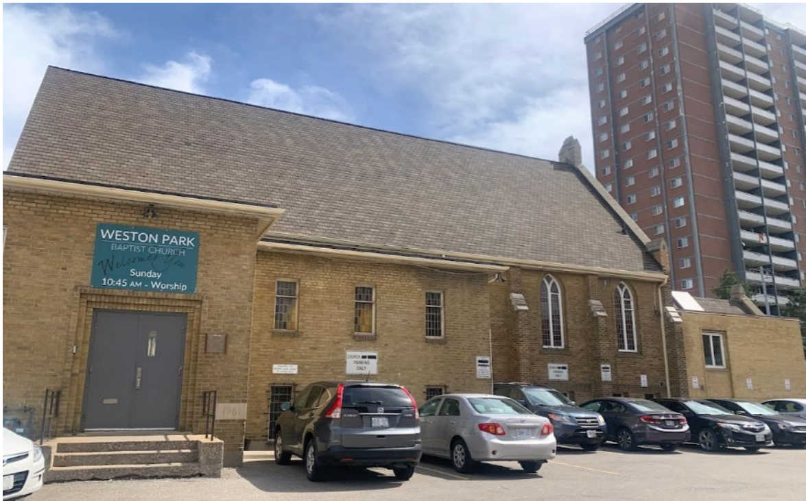
Image 34. North elevation and secondary entrance of the 1962 rear wing (Heritage Planning, 2023)
