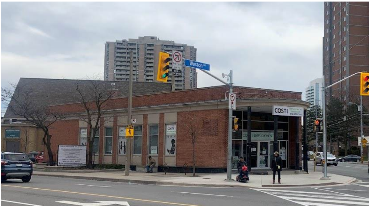
Image 44. Looking south at the main entrance and north elevation of the former Bank of Nova Scotia building. Note the limestone detailing with the cornice and large panels above and below the windows on the north and south elevations (Heritage Planning, 2023)
