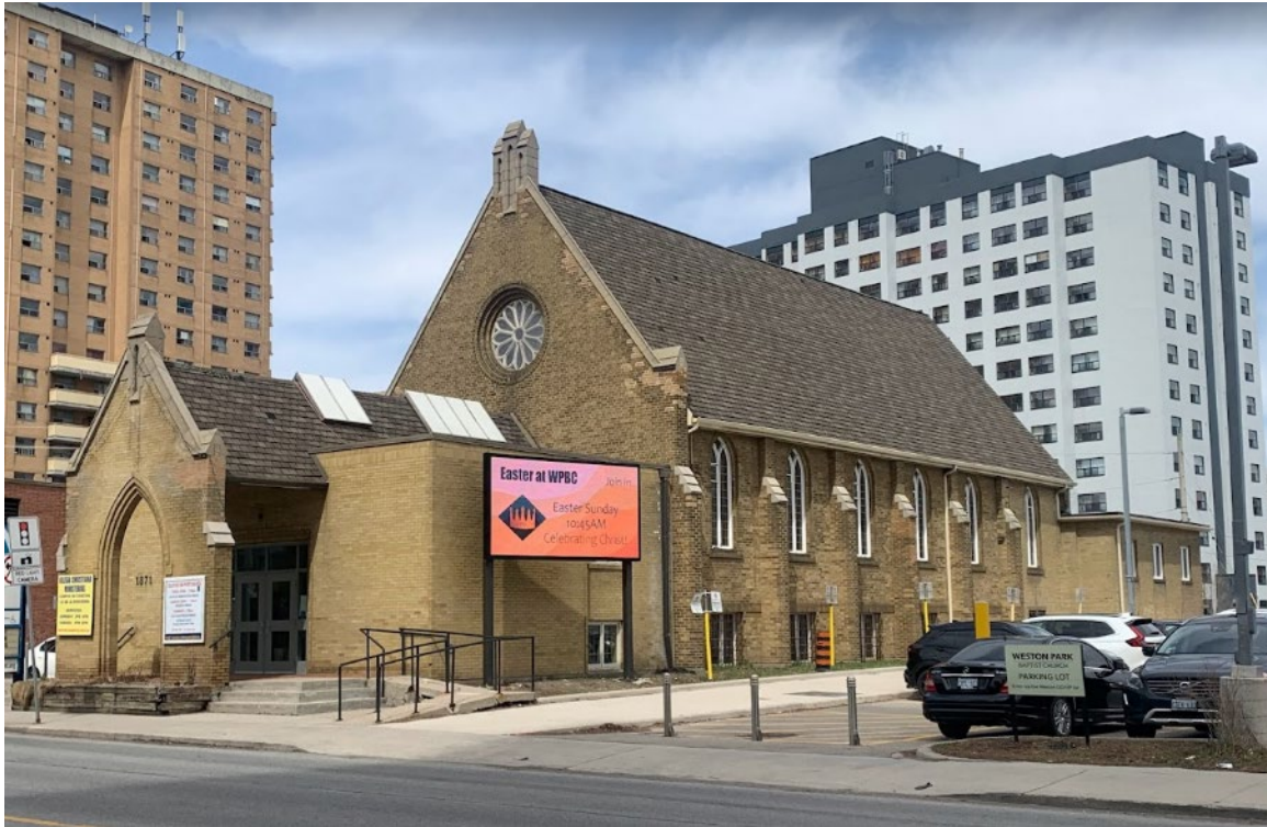
Image 30. Looking northeast at the south elevation of the church nave and 1983-1984 rectangular vestibule fronted by the reconstructed 1947 vestibule façade. (Heritage Planning, 2023)
