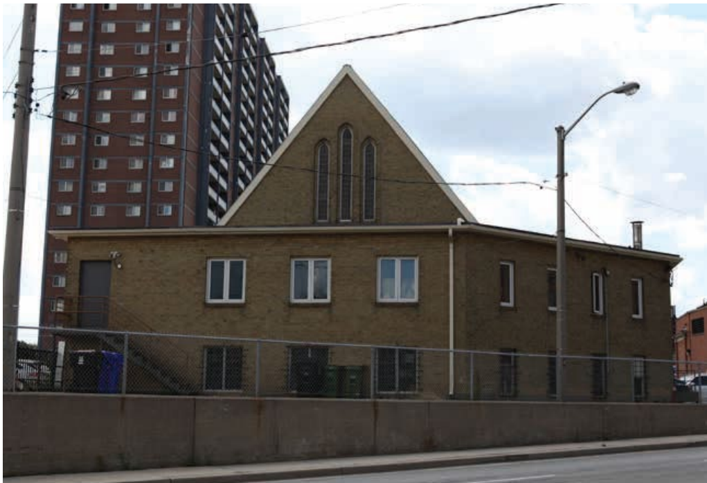
Image 36. Looking west at the 1962 rear wing and triple lancets in the east elevation of the sanctuary added in the same year. (ERA, 2021)
