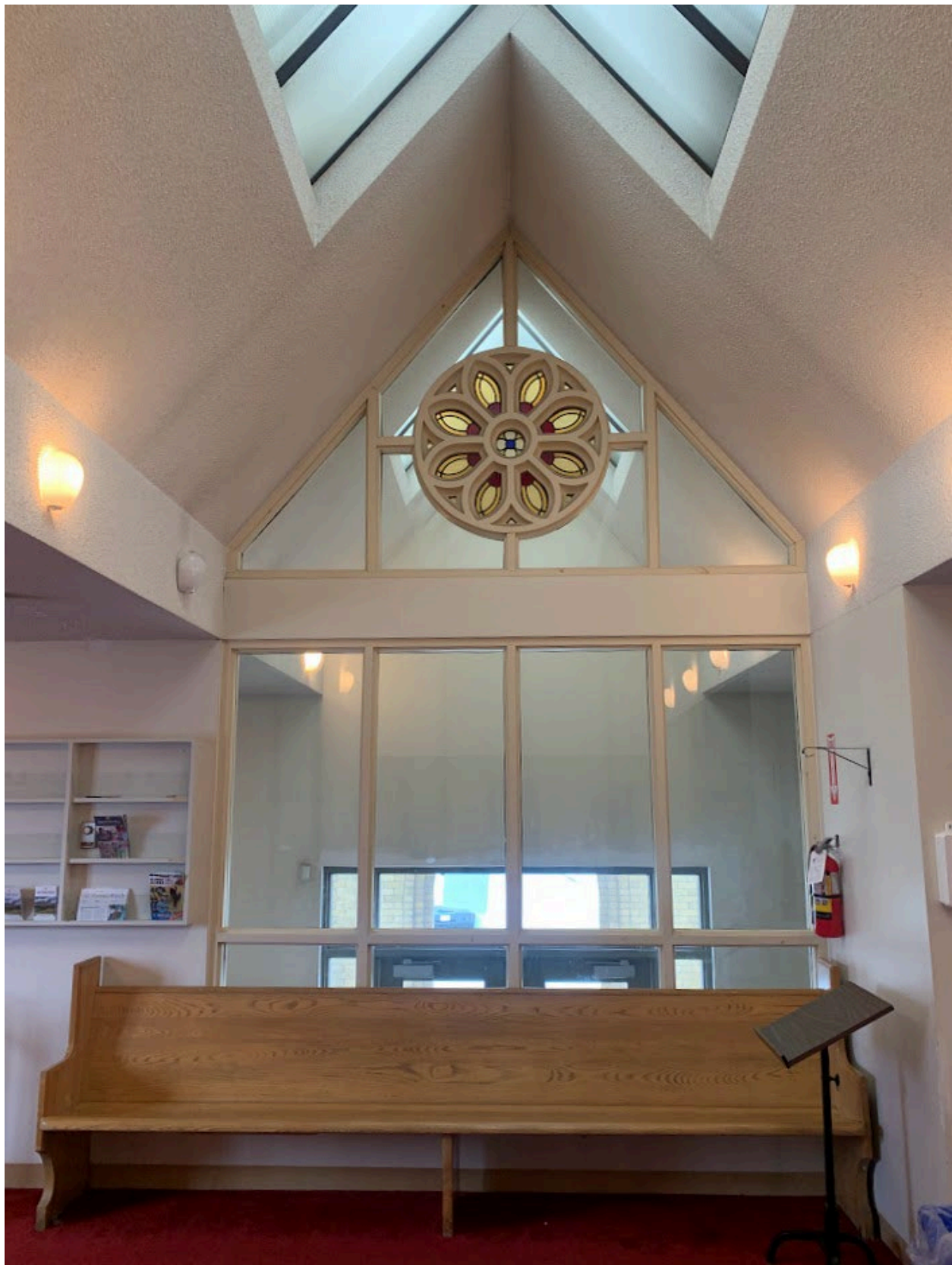
Image 37. Looking west from inside the 1983-1984 vestibule at the relocated rose transom originally located above the front entrance on the 1947 vestibule façade. (Heritage Planning, 2023)
