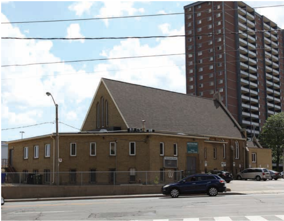
Image 35. Looking southeast across Lawrence Avenue West at the 1962 rear wing (ERA, 2021)
