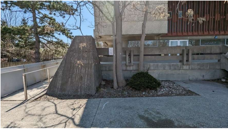
28. Northeast corner of the building showing the concrete pylon, 2023 (Heritage Planning)
