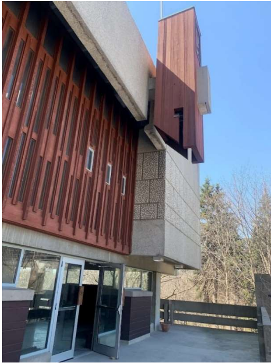
34. Current photo showing a detail of the wooden screen and west lantern on the north elevation, 2023 (Heritage Planning)
