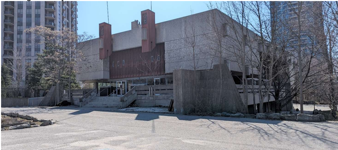
View of the subject property at 123 Wynford Drive, showing the west (principal) and south elevations of the former Japanese Canadian Cultural Centre (Heritage Planning, 2023).
