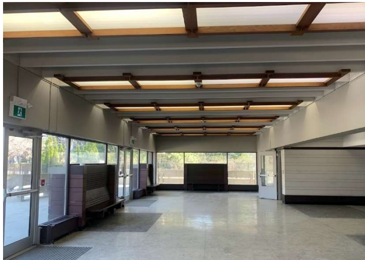
56. Current photo looking east across the lobby and showing the ceiling lighting and built-in bench seating along the exterior wall, d2023 (Heritage Planning)
