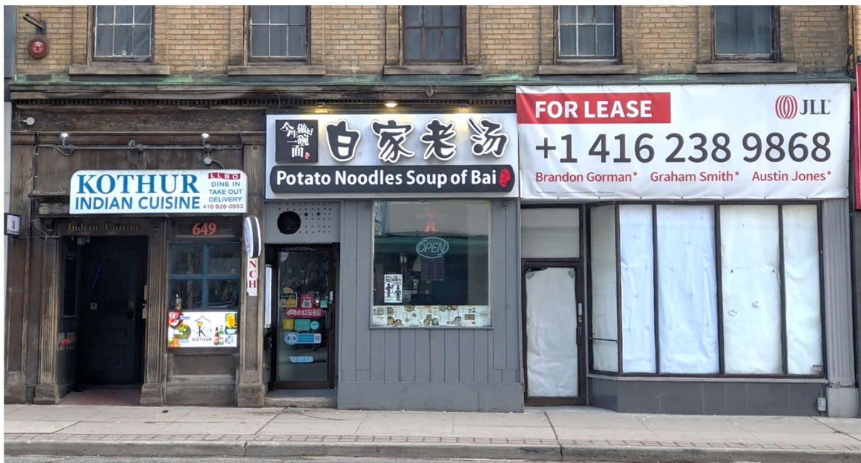
Figure 21. Detail of storefronts, west elevation of 649 Yonge Street (Heritage Planning, 2022).
