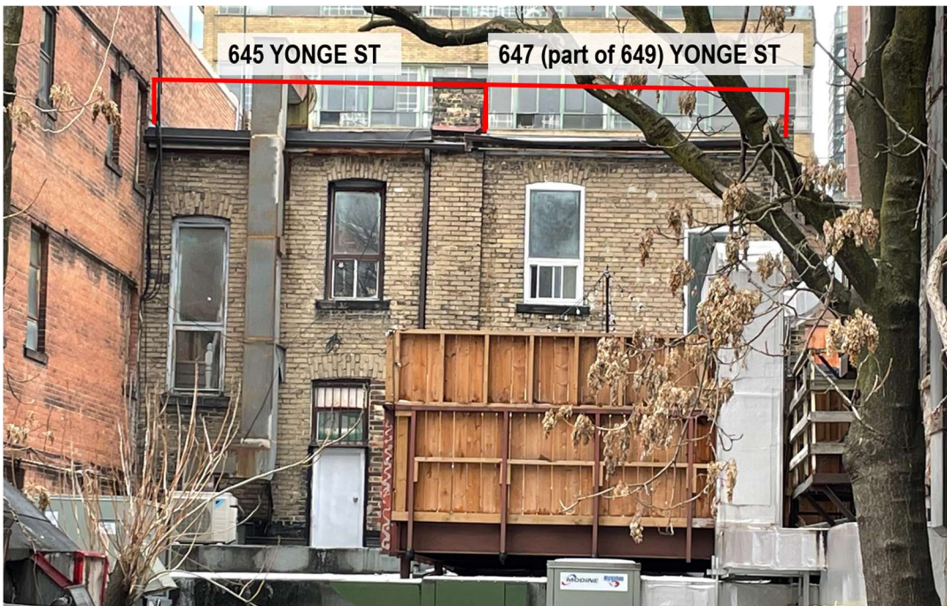
Figure 19. Rear (east) elevation of 645 and 649 Yonge Street. The portion of 649 Yonge Street that was historically 647 Yonge Street shares an exterior wall assembly with 645 Yonge Street, one of several indications that the buildings were constructed as a group (Heritage Planning, 2022).
