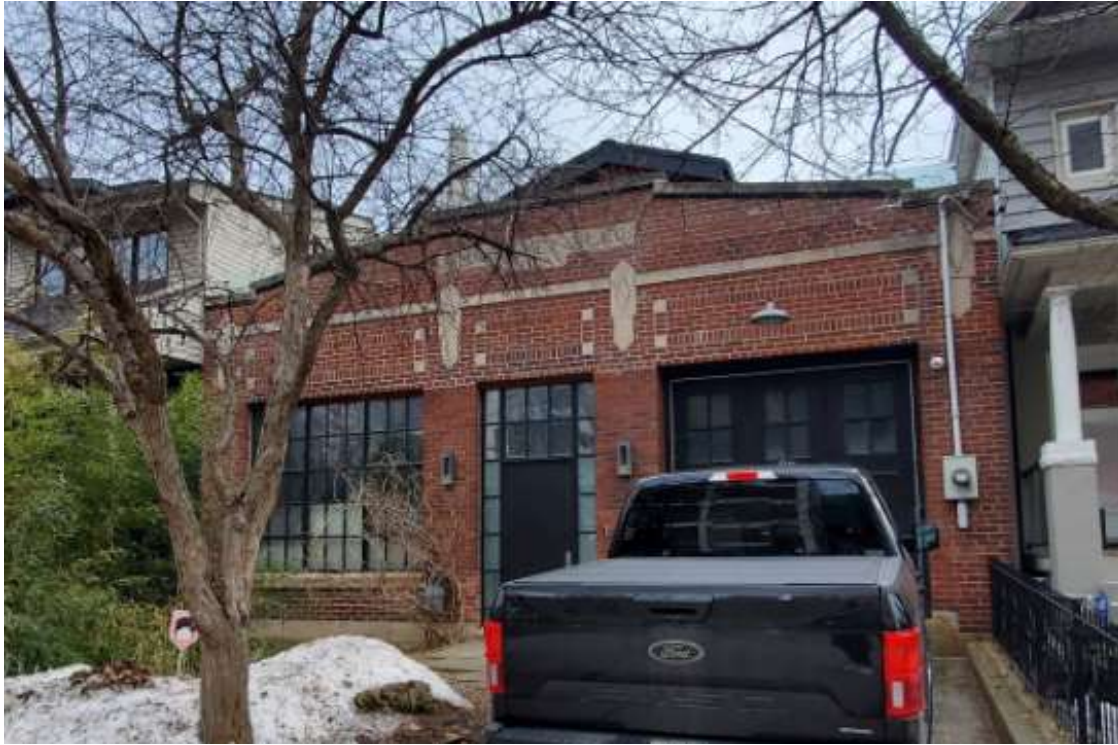
View of the principal (east) elevation of 87 Boston Avenue (Heritage Planning, 2022)
