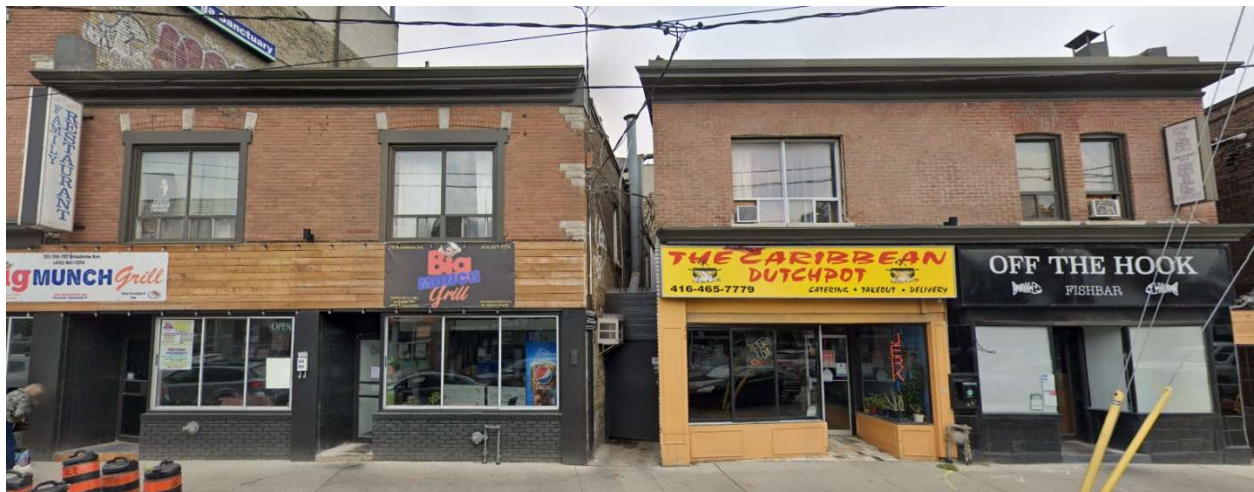
View of the principal (east) elevation of 749-753 Broadview Avenue (Heritage Planning, 2019)
