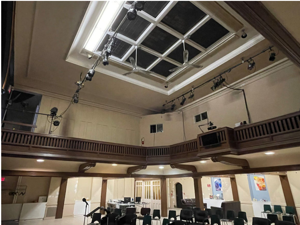
Figure 47: Auditorium of the Memorial Building showing the gallery balustrades and skylight, 2022 (City of Toronto Heritage Planning)
