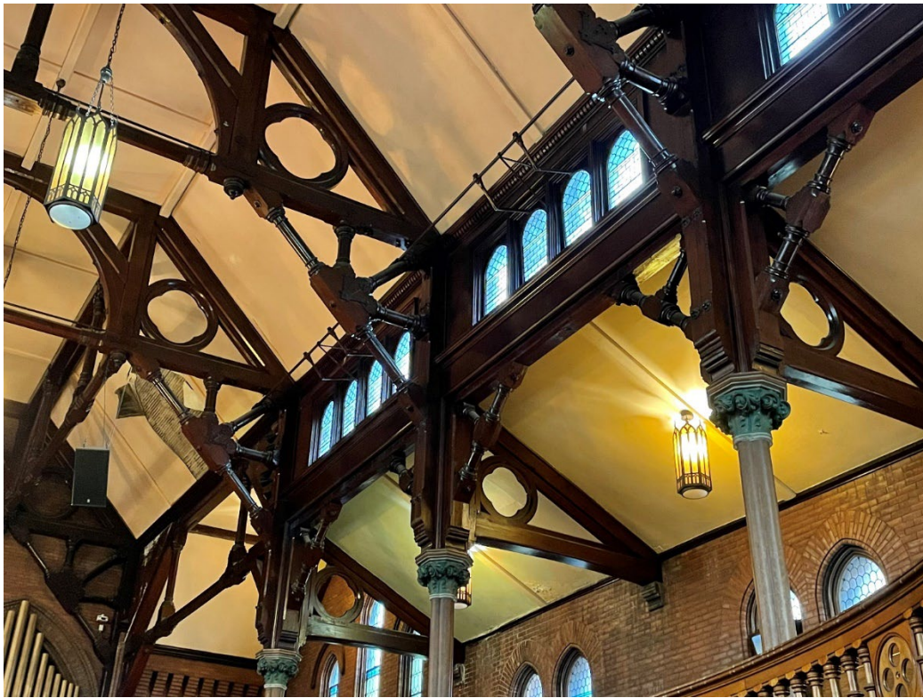
Figure 26: The ceiling of the Sanctuary showing the open, timber truss system, 2022 (City of Toronto Heritage Planning)
