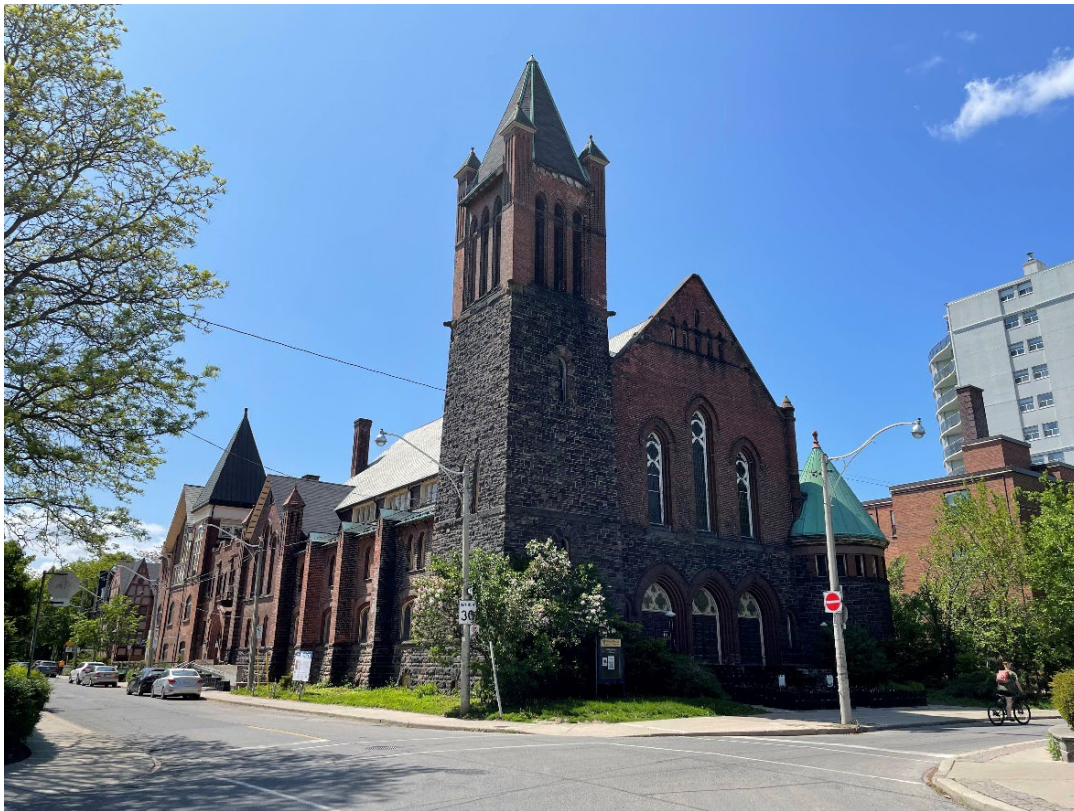
Figure 18: View of the front elevation of the Walmer Road Baptist Church at the southeast corner looking west along Lowther Street. 2023 (Heritage Planning)
