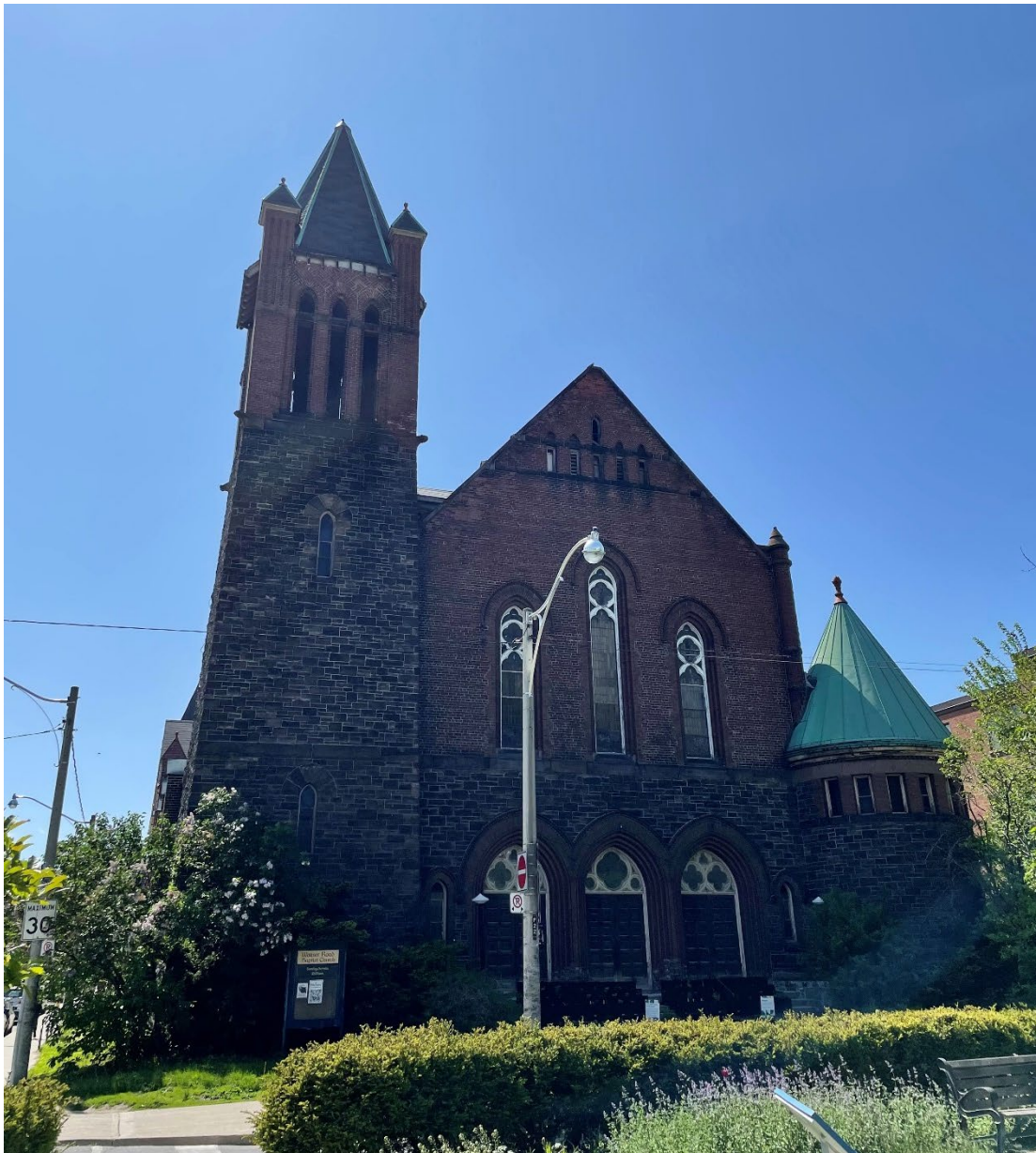
Walmer Road Baptist Church, front (East) elevation, 2023 (Heritage Planning)
