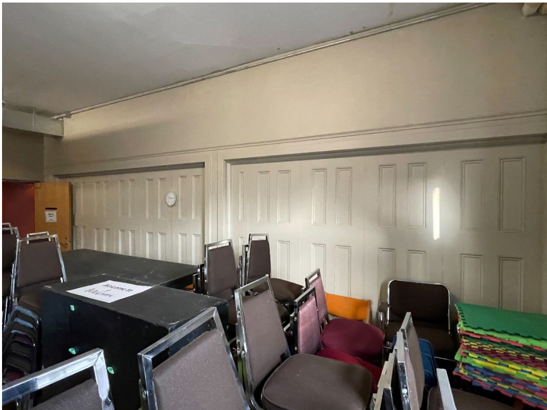
Figure 49: An example of the sets of sliding doors creating flexible classroom space
