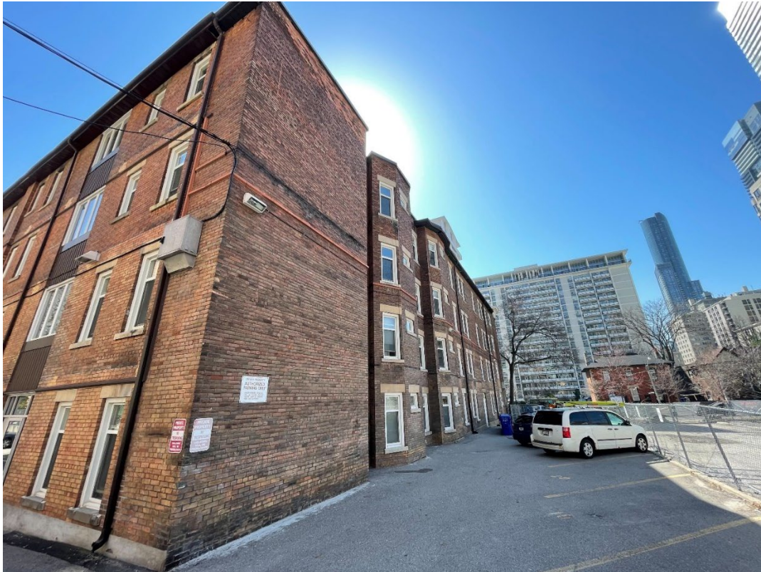
Figure 10: West façade of 36 Maitland Street, viewed from the north, 2023 (Heritage Planning)
