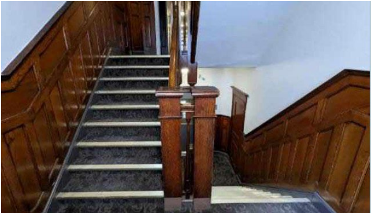
Figure 14: Main staircase and lobby of 42 Maitland Street, 2022 (Heritage Impact Assessment, LHC Planning and Architecture, December 22, 2022)
