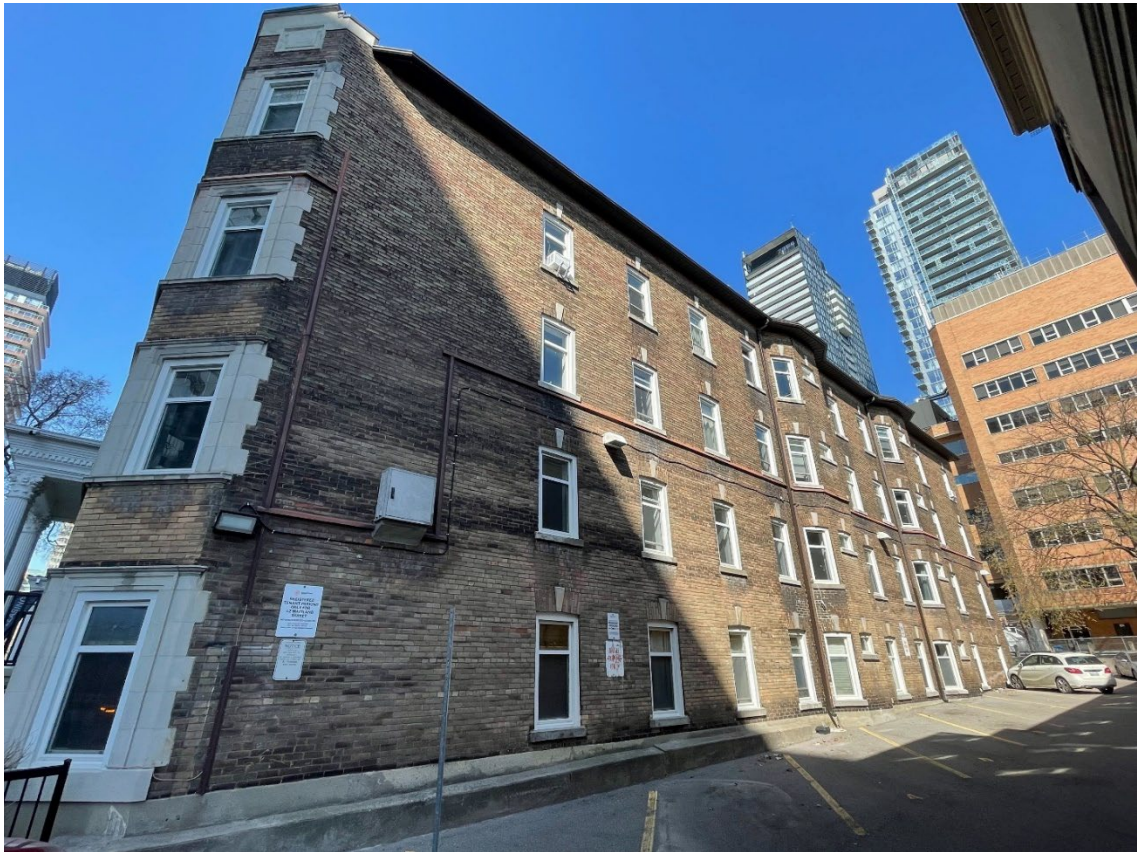
Figure 8: East façade of 42 Maitland Street, 2023 (Heritage Planning)
