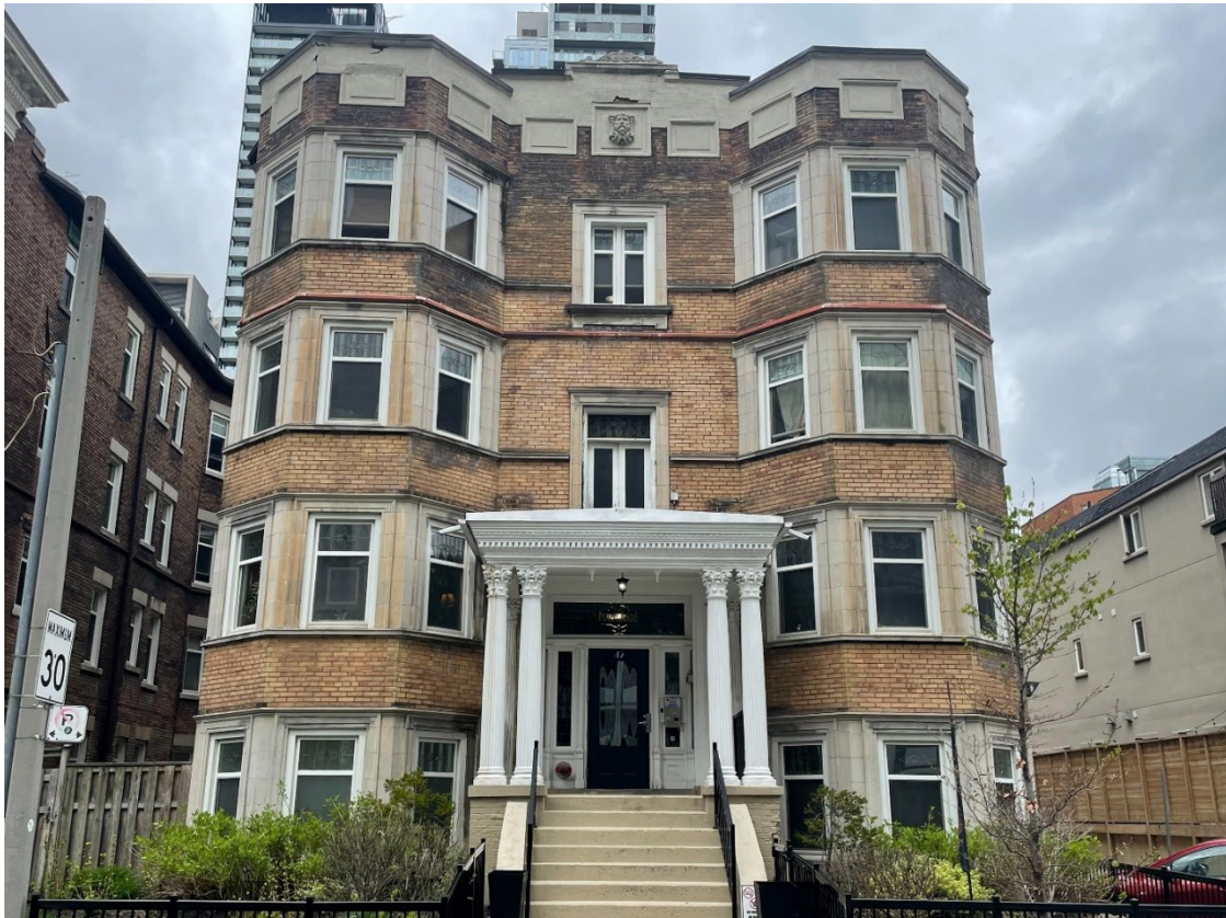
Figure 6: South (main) façade of 42 Maitland Street, 2023 (Heritage Planning)
