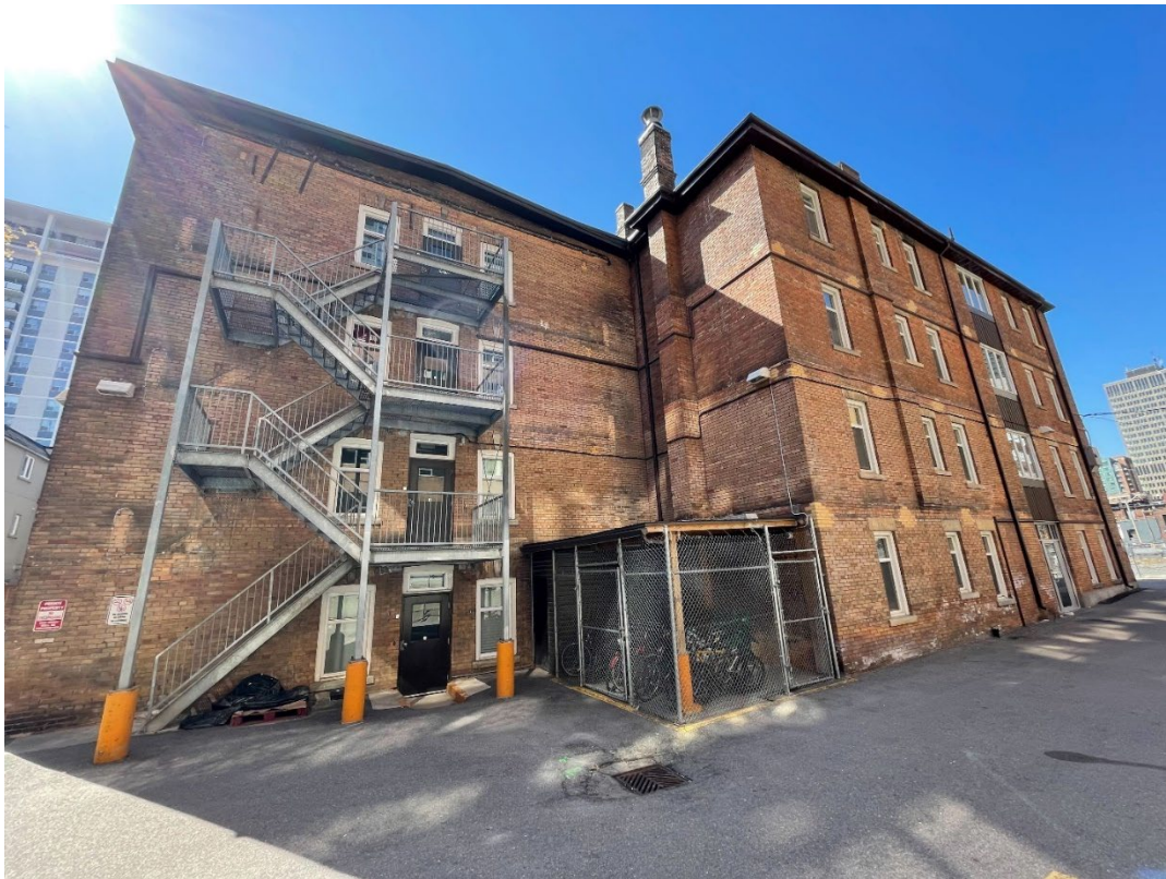
Figure 9: North (rear) façades of 36 (right) and 42 Maitland Street (left), 2023 (Heritage Planning)
