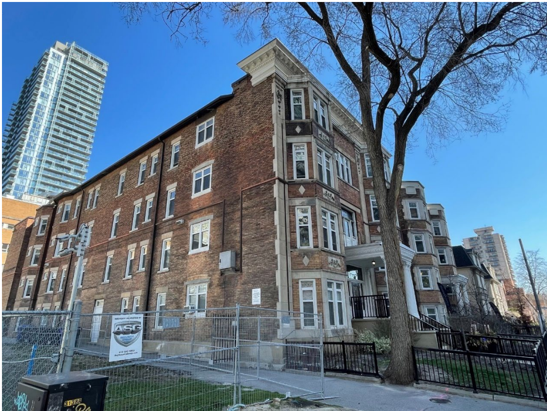
Figure 11: West façade of 36 Maitland Street, viewed from the south, 2023 (Heritage Planning)
