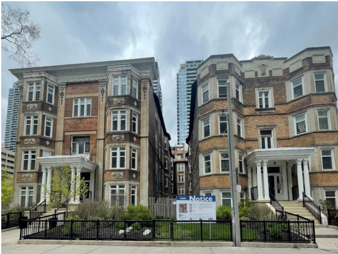
Figure 7: South (main) façades of 36 and 42 Maitland Street, 2023 (Heritage Planning)
