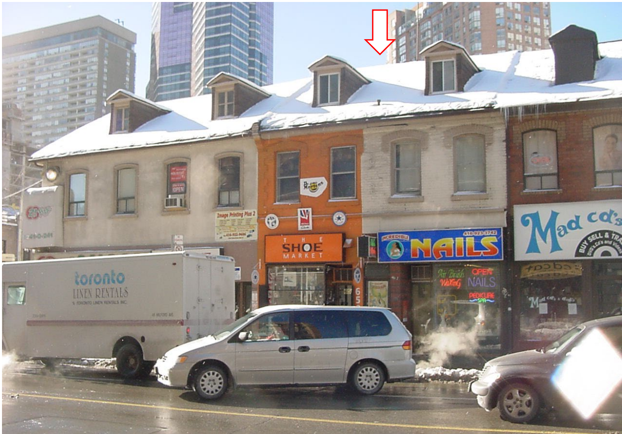
Figure 7. Photograph from 2004, showing 646-654 Yonge Street (Heritage Planning, 2004). 650 Yonge Street is indicated by the arrow.
