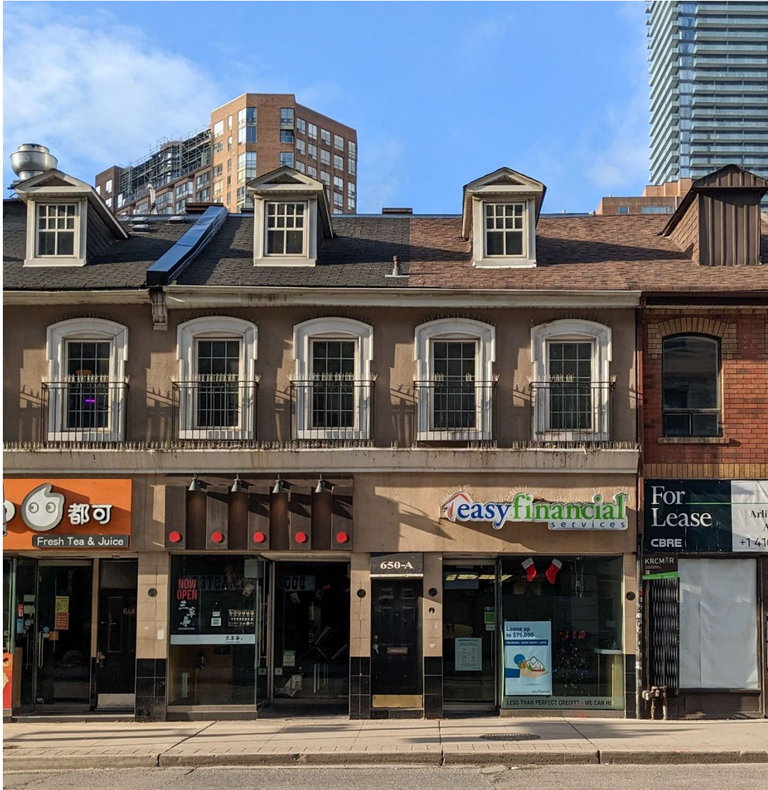
Figure 9. Primary (east) elevation of 650 Yonge Street (Heritage Planning, 2023)
