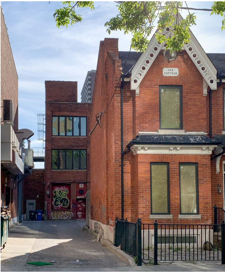
Figure 17. West elevation of 680 Yonge Street as viewed from St Nicholas Street, with one of the Scottish Ontario and Manitoba Land Company Cottages visible on the right (Heritage Planning, 2023).
