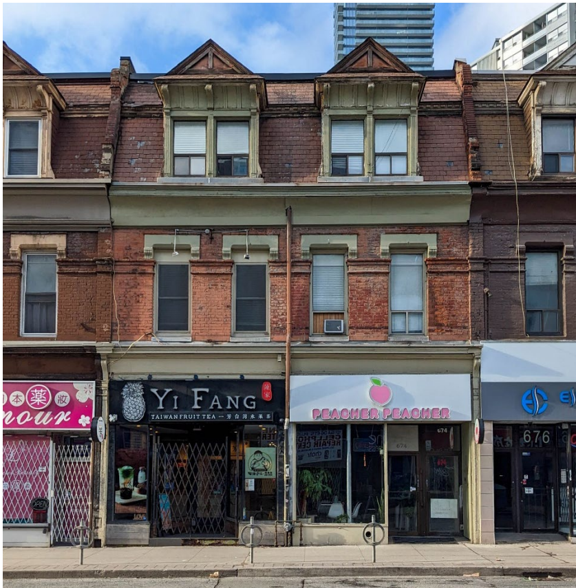
Figure 11. Primary (east) elevation of 672 Yonge Street (Heritage Planning, 2023).
