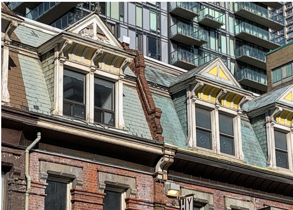
Figure 14. Detail of dormers, 678-680 Yonge Street (Heritage Planning, 2023).
