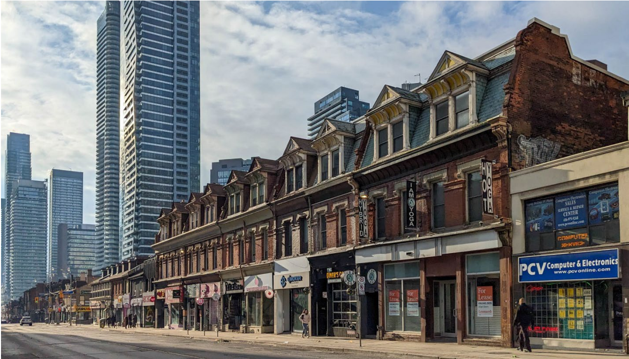
View of the subject properties at 664-680 Yonge Street, looking southwest (Heritage Planning, 2022)
