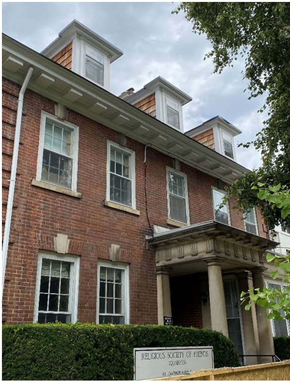
Figure 12. South or principal elevation showing a largely symmetrical composition characteristic of the Georgian Revival style. (Heritage Planning, 2023)
