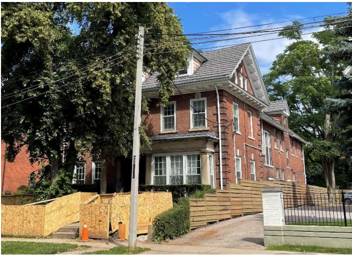
Figure 16. South and east elevations. (Heritage Planning, 2023)
