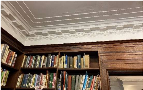
Figure 19. Dentils on covered ceiling. (Heritage Planning, 2023)
