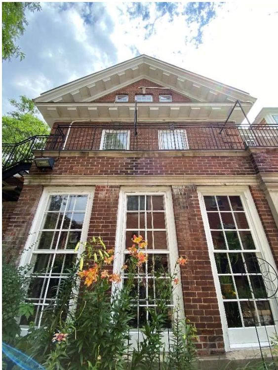
Figure 14. West elevation showing elongated window bays, dentils on gable end, and symmetry (Heritage Planning, 2023)
