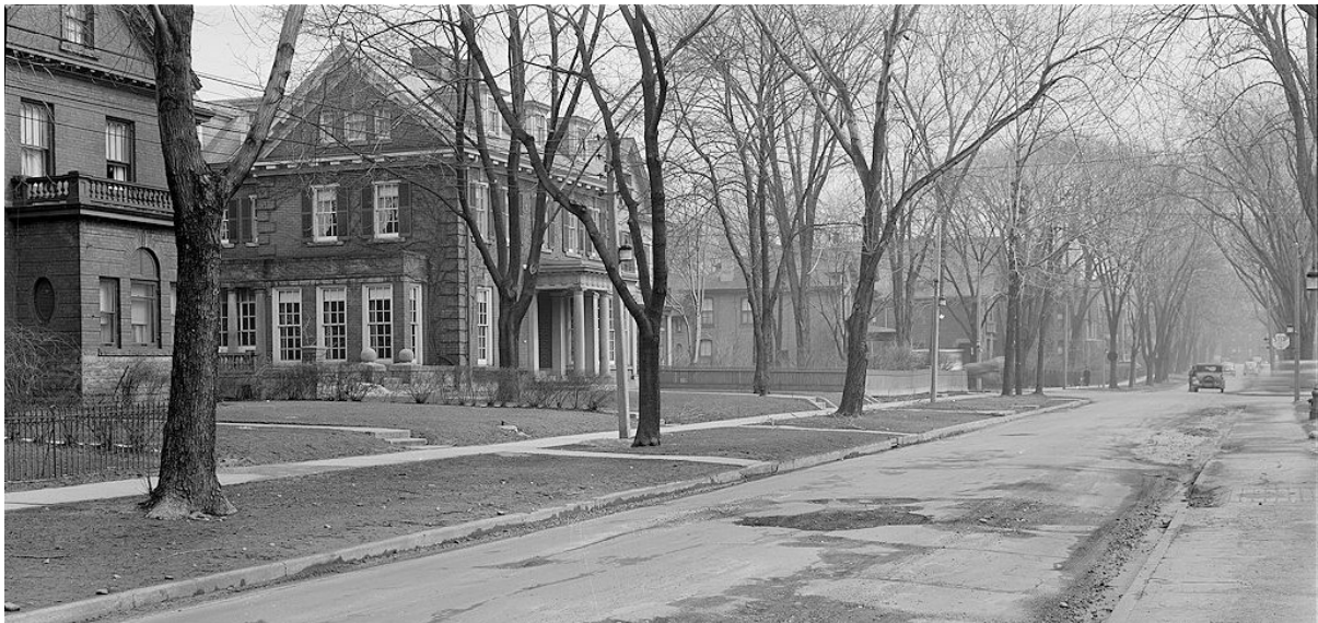
Figure 6. The property at 60 Lowther Avenue showing the south and partial view of the west elevations. The property is set back from the public realm with a lawned front yard. A partial view of the narrow pathway and masonry gateway is shown. (City of Toronto Archives, 1941)
