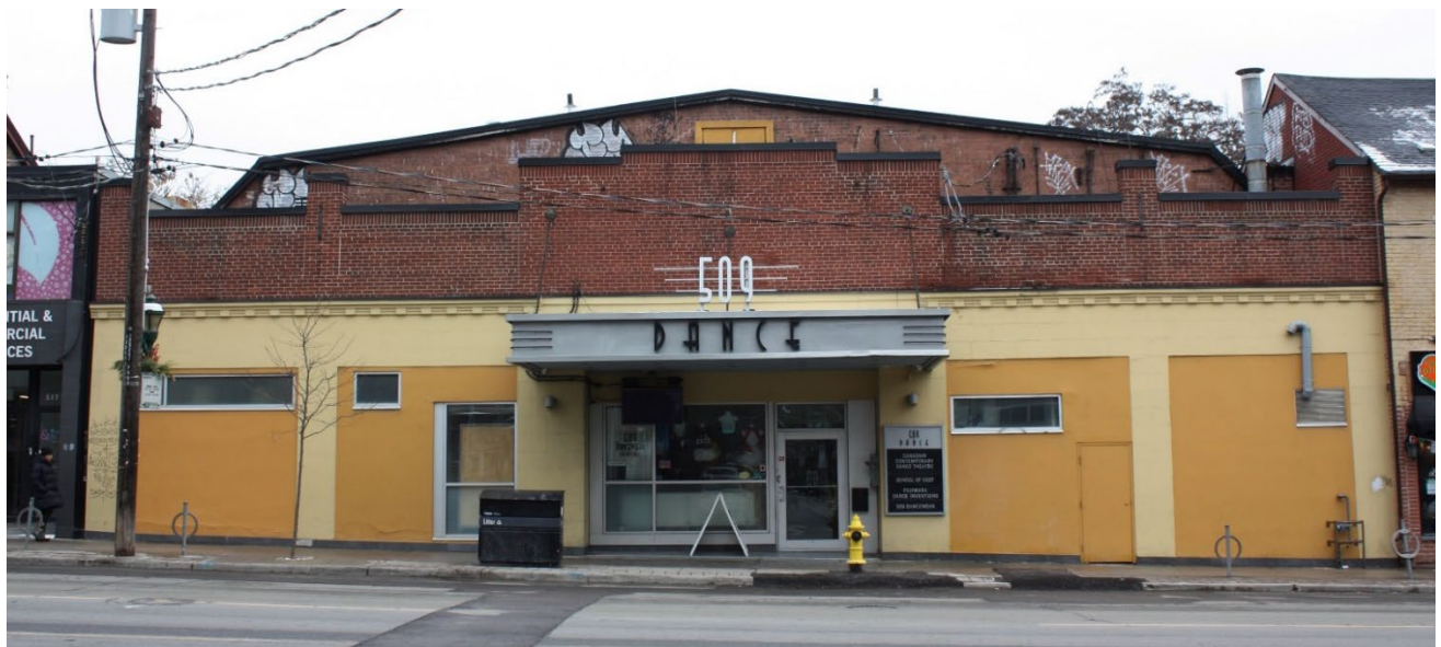
Figure 1. Main elevation (west) of subject property, facing onto Parliament Street (Heritage Planning, 2023).
