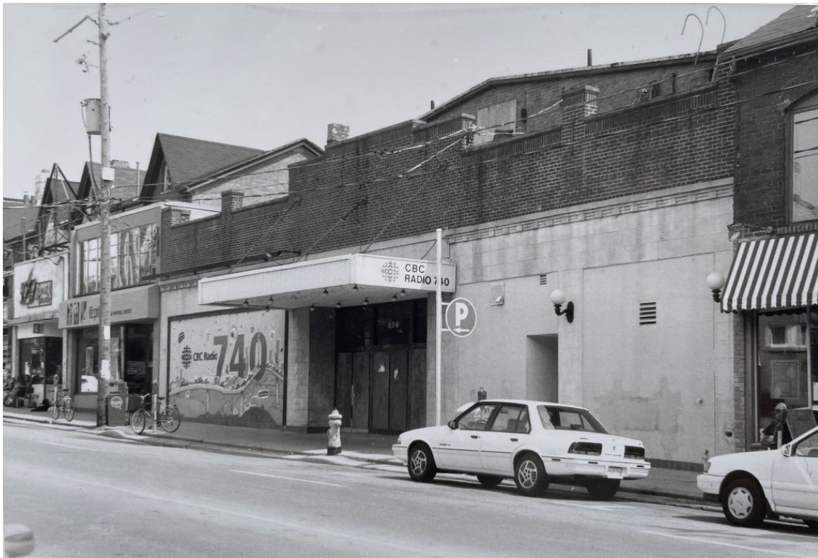
Figure 10. Exterior photo of 509 Parliament Street's main facade (west) during CBC's ownership, 1980s. Note the infill of the original shopfronts, and the alterations to the marquee signage (City of Toronto Archives).
