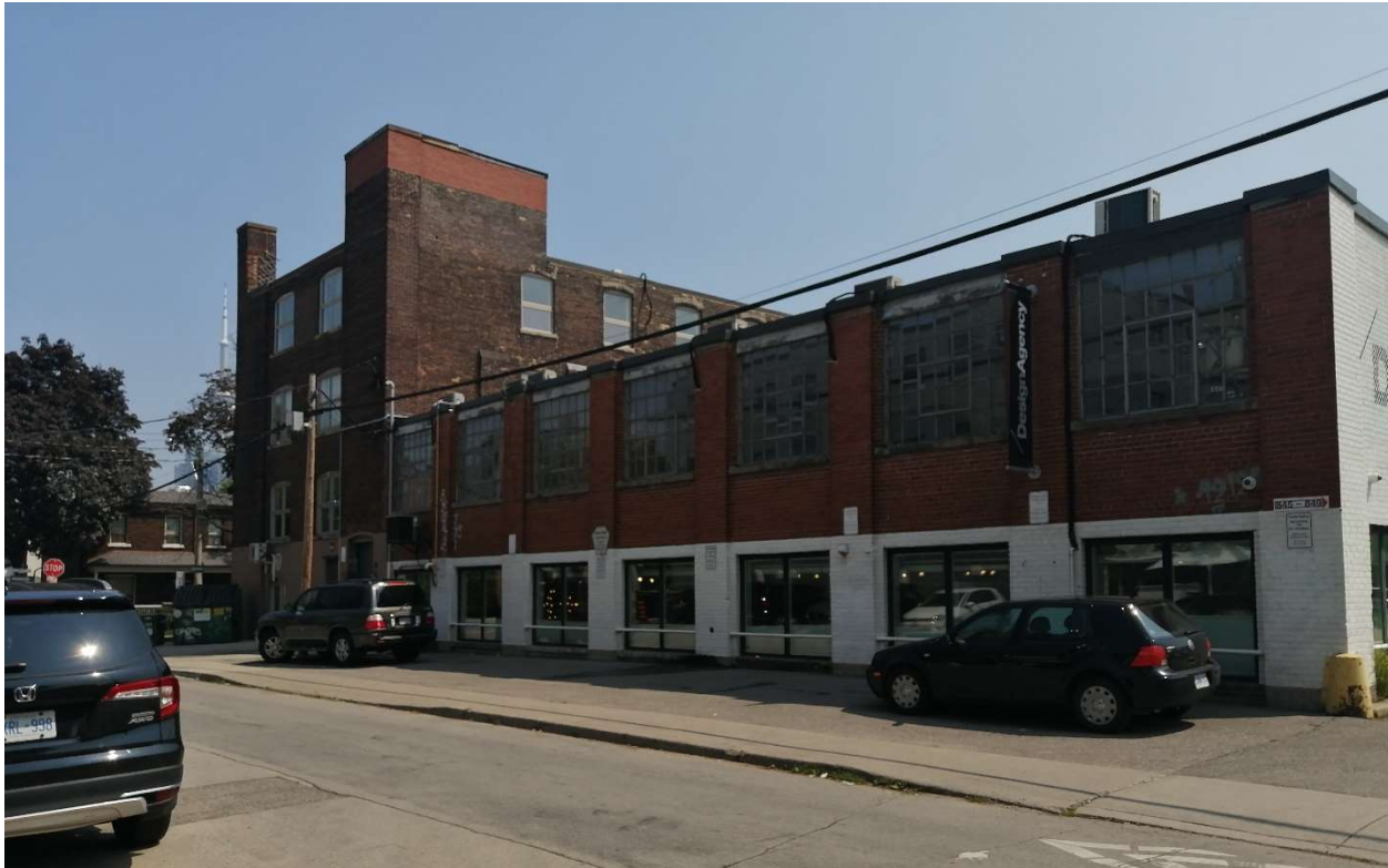
Figure 24: Early 20th century industrial building at 72-74 Stafford Street (Heritage Planning, 2023).
