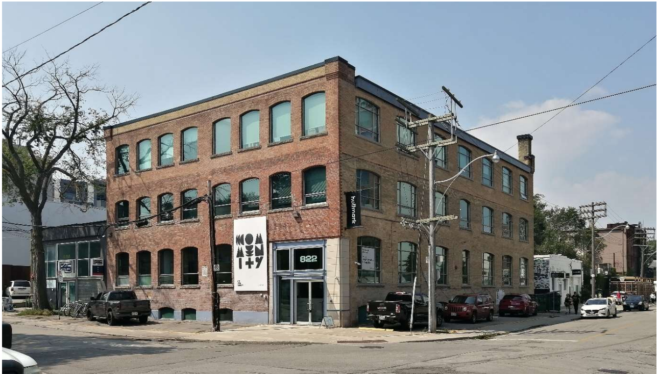
Figure 1: 822 Richmond Street West (Heritage Planning, 2023).
