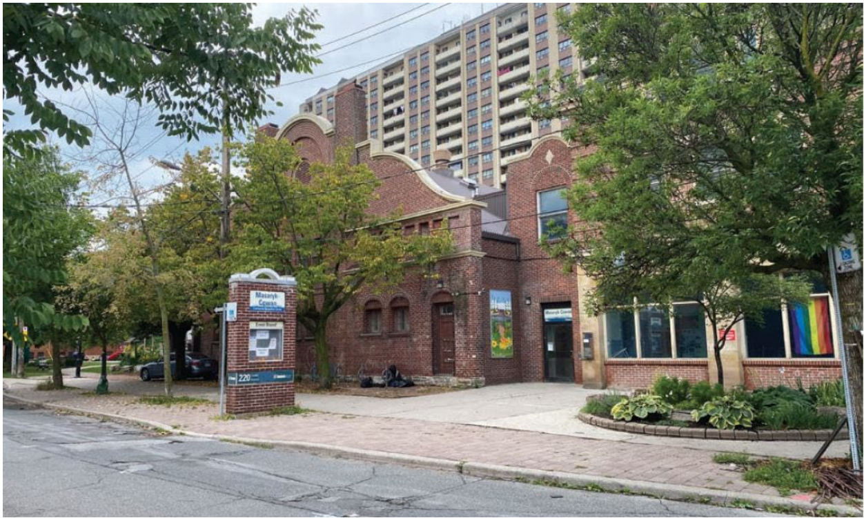
Principal (east) elevation of the entirety of 220 Cowan Avenue (ERA Architects Inc., 2022).
