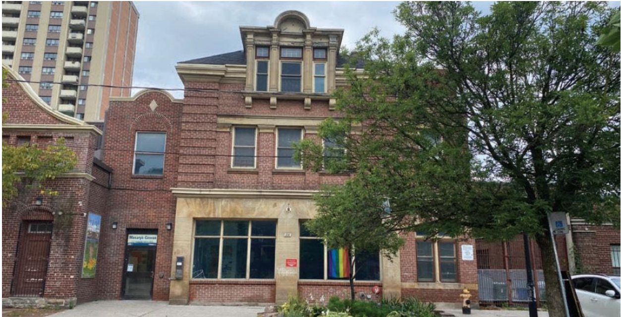
Principal (east) elevation of the former Fire Hall No.18 at 220 Cowan Avenue (ERA Architects Inc., 2022).
