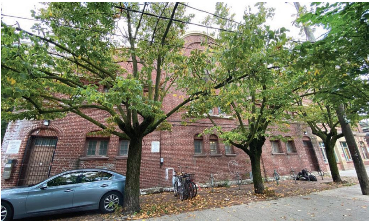
Principal (east) elevation of the former Parkdale Curling Club at 220 Cowan Avenue (ERA Architects Inc., 2022).
