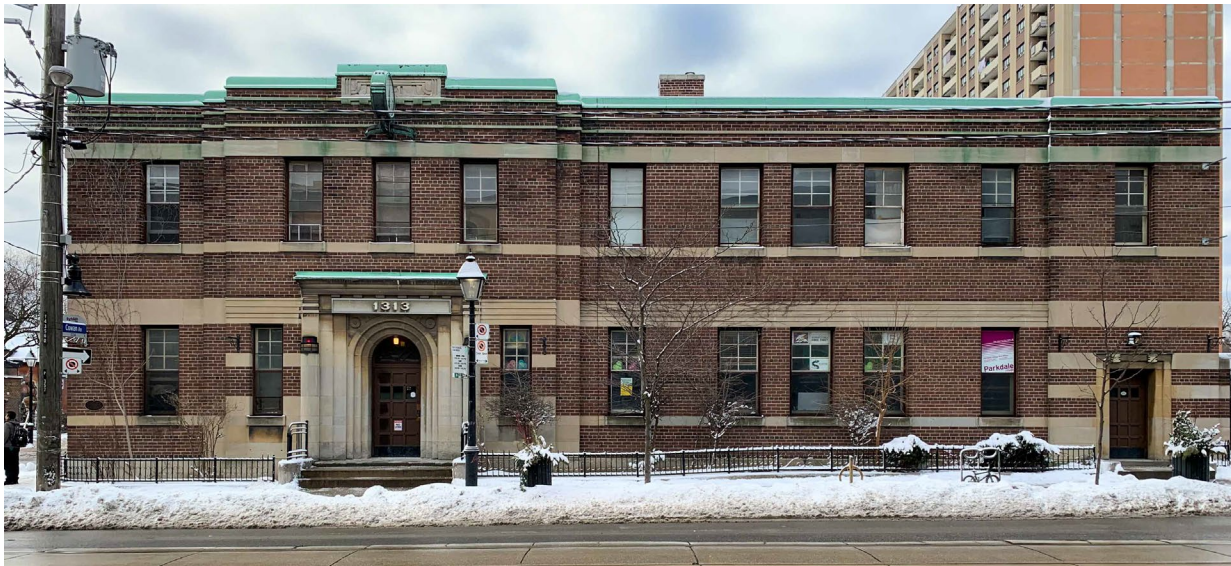
Principal (north) elevation of 1313 Queen Street West (Heritage Planning, 2023).
