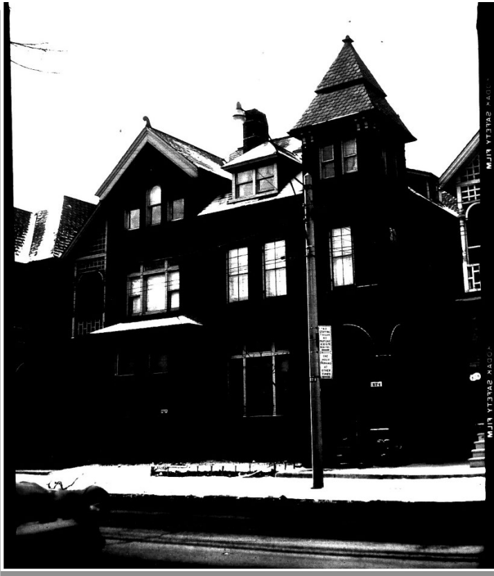
Figure 4 1957 image of the east elevations of 572 and 574 Sherbourne Street (City of Toronto Archives).
