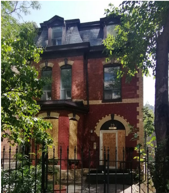
Figure 21 North elevation of 29 Linden Street (Heritage Planning, 2023).
