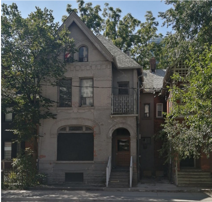
Figure 12 570 Sherbourne Street showing deeply recessed "tail" connecting to 572 Sherbourne Street to the north (Heritage Planning 2023).
