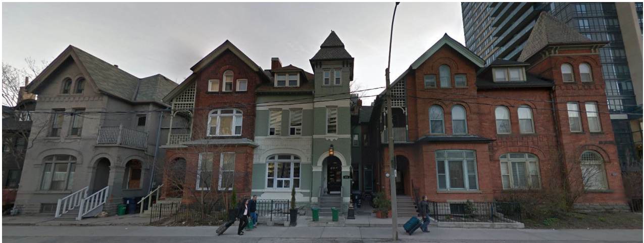
Figure 8 East elevations of 570-576 Sherbourne Street and 37 Linden Street (Google, April 2015).
