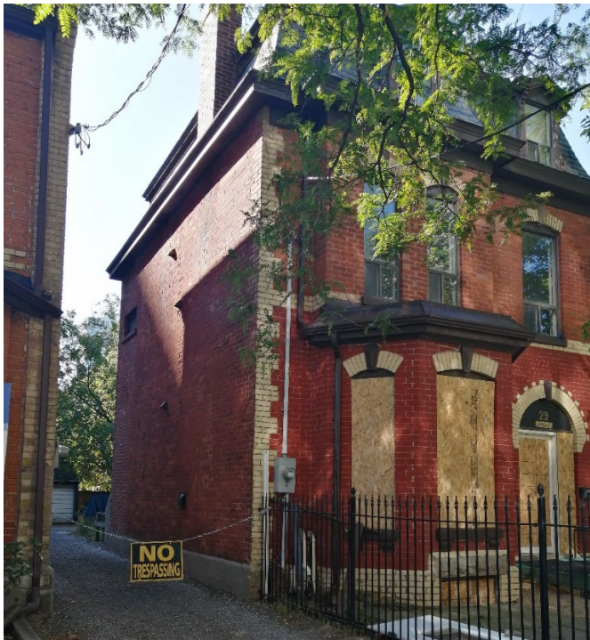
Figure 23 East and north elevations at 29 Linden Street (Heritage Planning, 2023).
