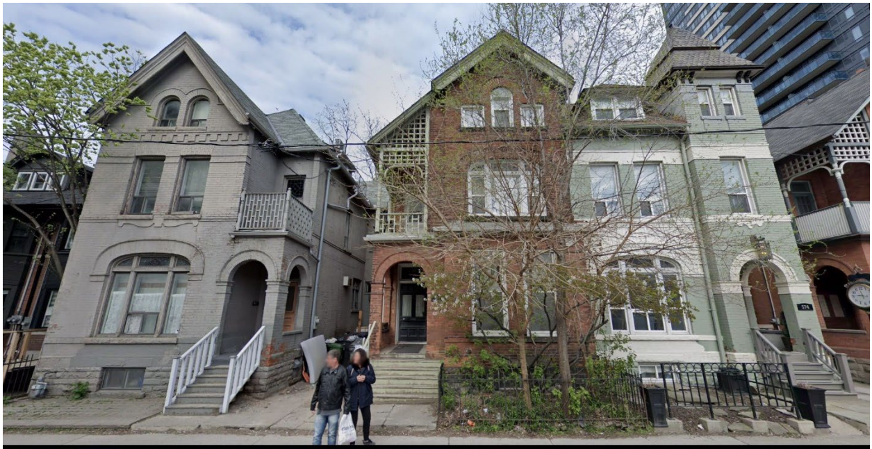
Figure 11 570, 572, and 574 Sherbourne Street (Google, May 2019).
