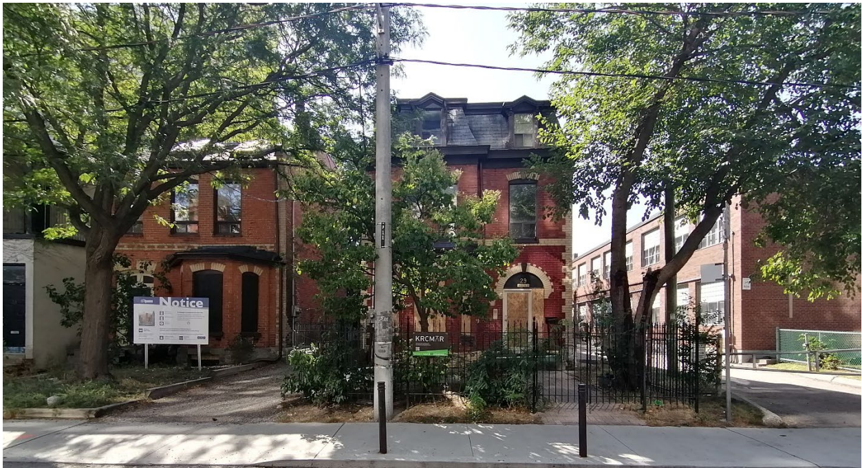
Figure 29 Looking south towards 29 Linden Street and adjacent properties (Heritage Planning, 2023).
