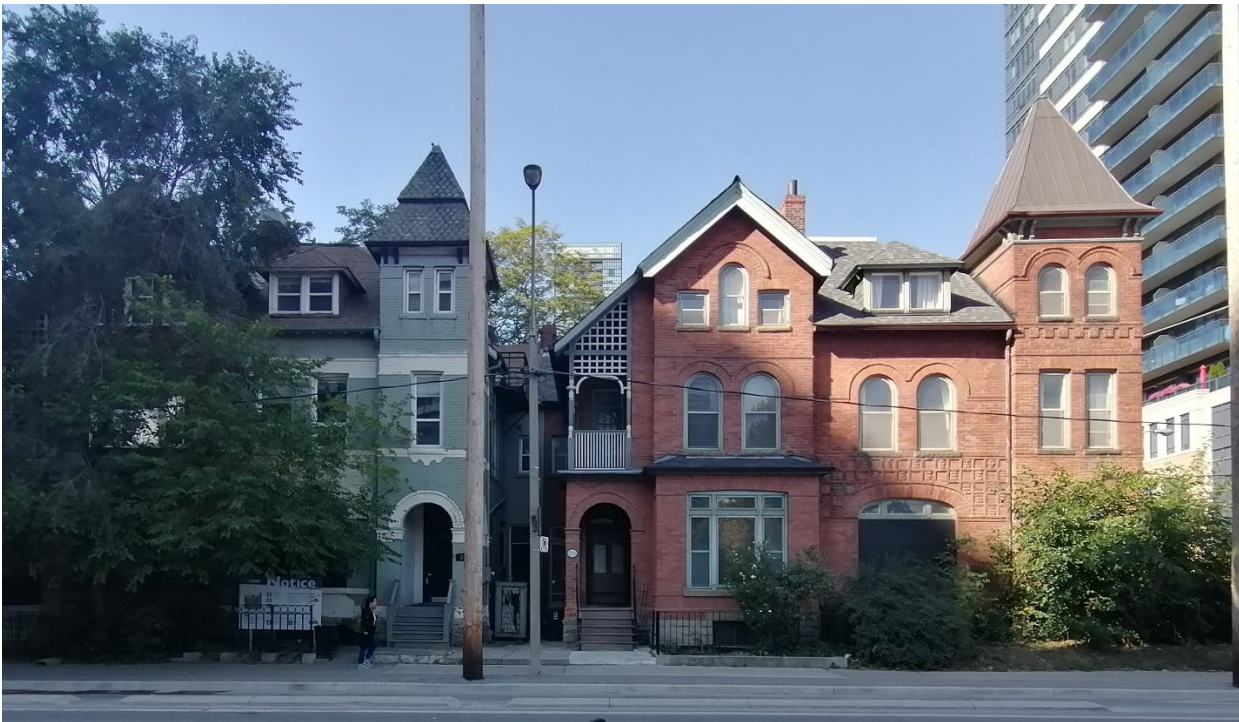
Figure 14 572-576 Sherbourne Street and 37 Linden Street showing deeply recessed "tail" connecting 574 and 576 Sherbourne Street (Heritage Planning, 2023).
