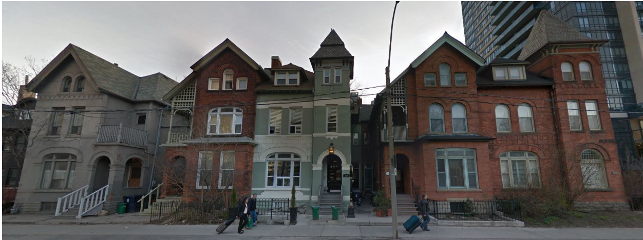
An unobstructed view of 570, 572, 574 and 576 Sherbourne Street (Google, April 2015)
