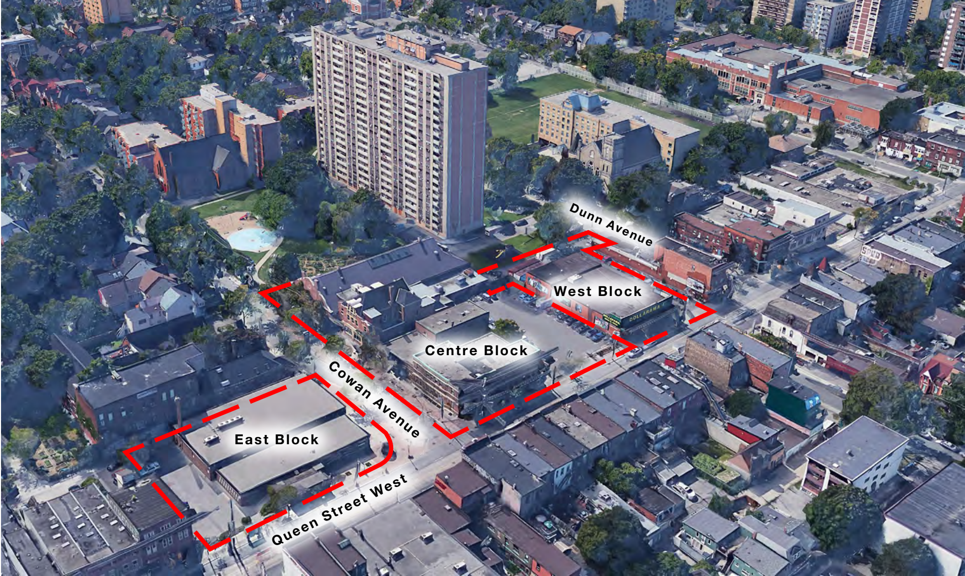
Figure 6 / Parkdale Hub today: aerial view (2020).
