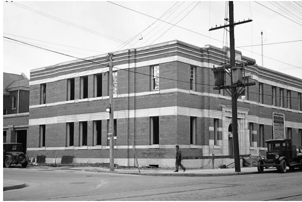
Figure 12 / Historic view of north and east elevations (C.1931).
