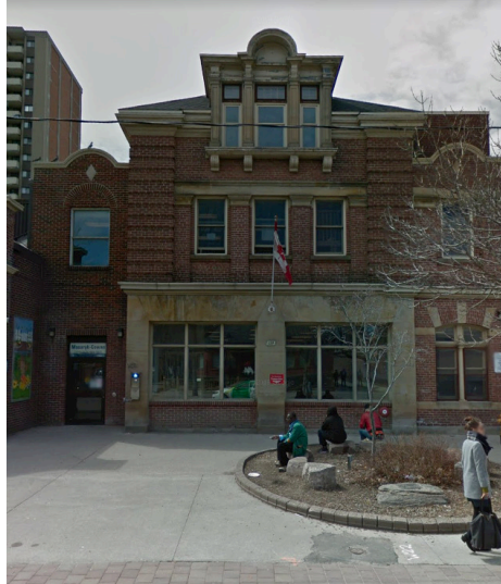
Figure 21 / 220 Cowan Avenue Today: Principal (east) façade of Fire Hall No.18 (2020)
