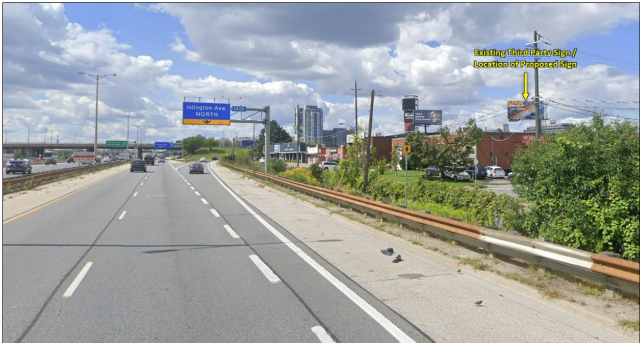
Figure 1: Looking northwest from F.G. Gardiner Expressway to the Premises
