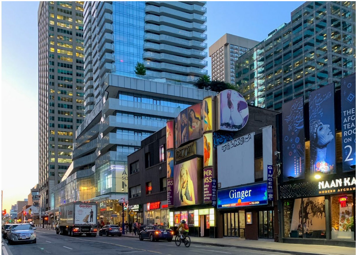
Figure 18. 699 and 707 Yonge Street, viewed from the southwest (Heritage Planning, 2023).
