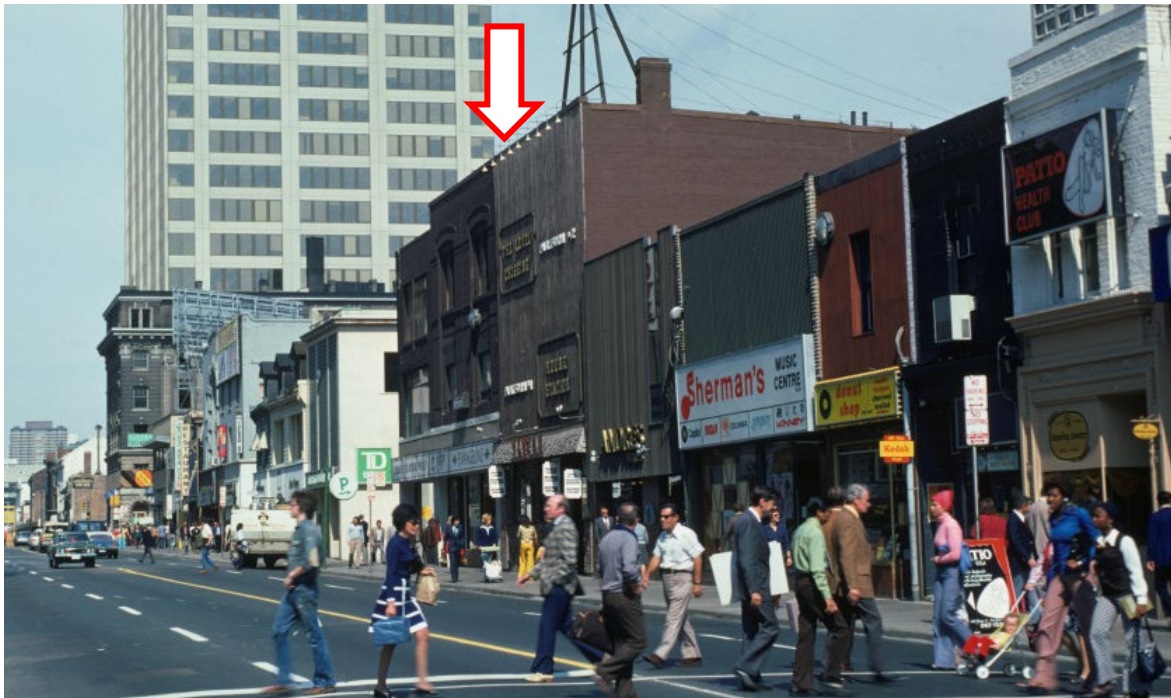
Figure 14. Archival photograph from 1974, showing the wood siding on 699 Yonge Street. The northern half of the row building (entrances at 703-705 Yonge Street) has not yet been over-clad (City of Toronto Archives, Fonds 1526, File 2, Item 8).
