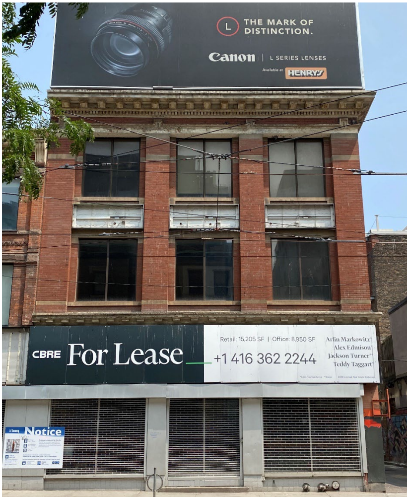
13. West (principal) elevation of 119 Church Street, adjacent to Ditty Lane, a public laneway (Heritage Planning, 2023)
