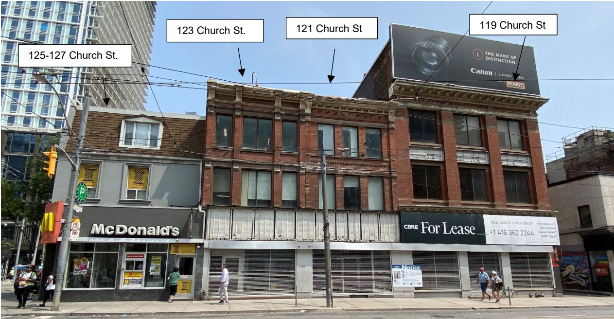
Figure 1: 127 Church Street (including entrance addresses 125, 123 and 121 Church Street) and 119 Church Street. NOTE: The structure (125 Church Street) shown on the left and located on the corner property at 127 Church Street is not a heritage attribute (Heritage Planning, 2023)
