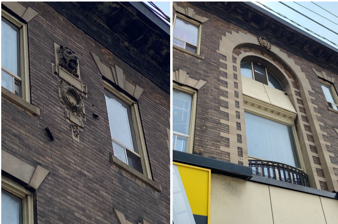
25. (left) and 26. (right) Architectural details in stone, buff-brick cladding in Don Valley brick, prominent metal cornice painted in black (Heritage Planning, 2023)
