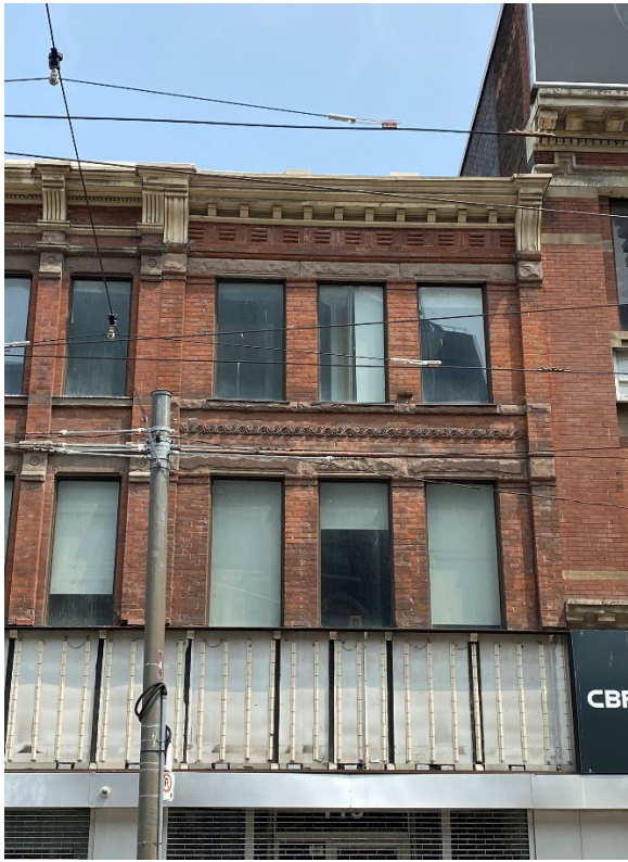
16. West (principal) elevation of entrance address 121 Church Street showing a late-Victorian architectural style (Heritage Planning, 2023)
