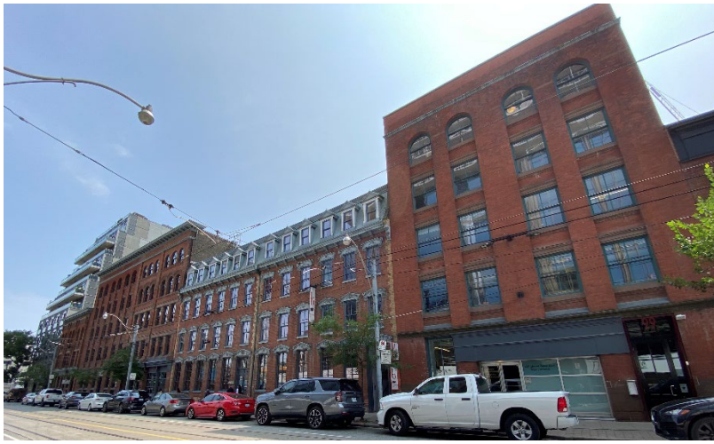
27. Robertson Brothers industrial complex at 99 - 123 Queen Street East, designated under Part IV of the OHA (Heritage Planning, 2023)
