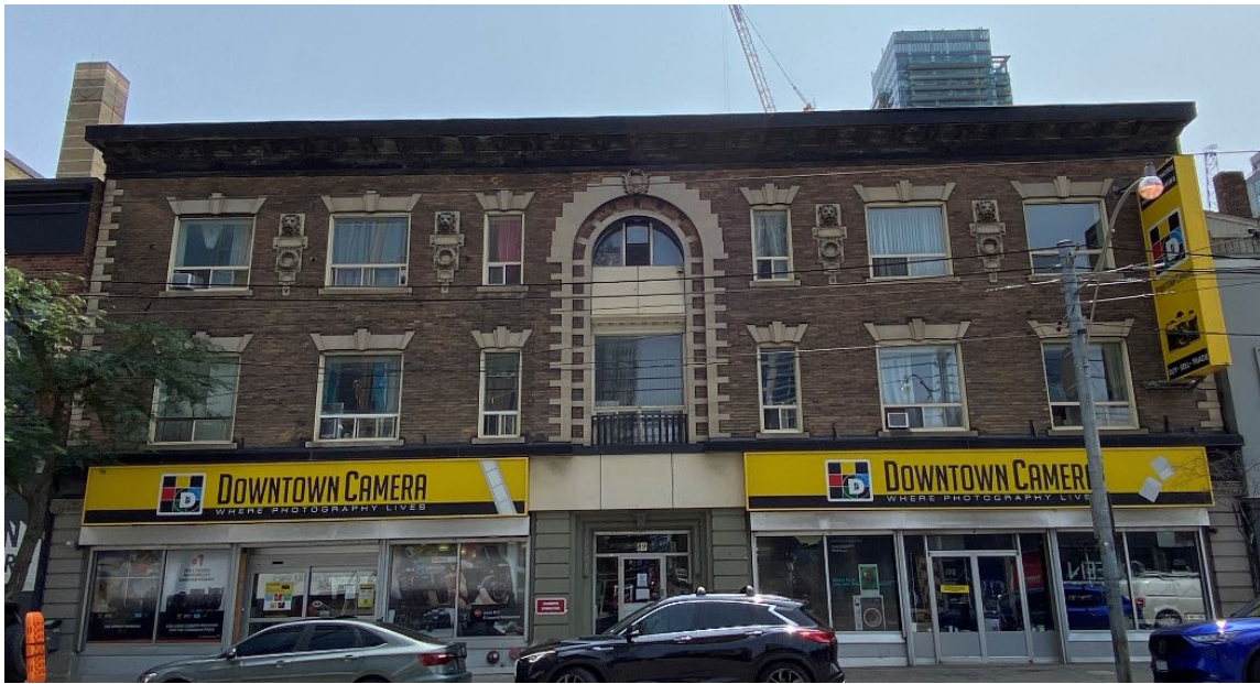
24. Front elevation of 89 Queen Street East showing Edwardian Classicism architectural elements (Heritage Planning, 2023)
