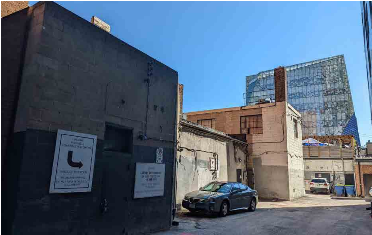
Figure 25: South elevation (ERA, 2022).
