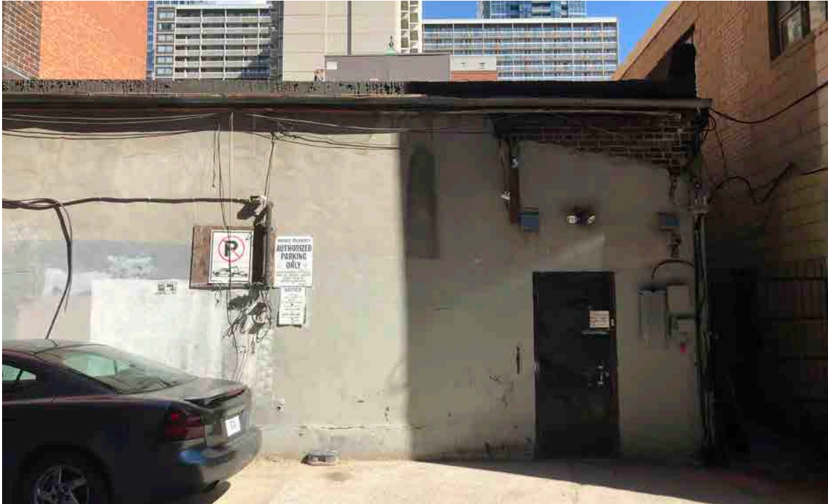
Figure 24: The Eastern portion of the south elevation (ERA, 2022).
