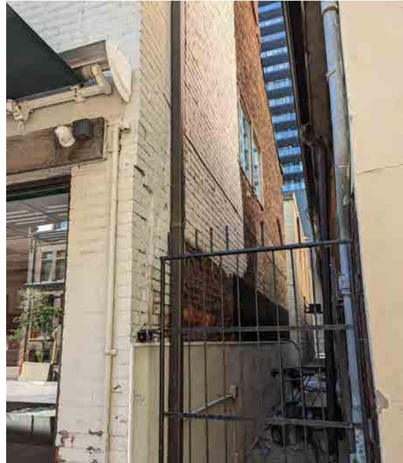
Figure 18: West elevation (ERA, 2022).
