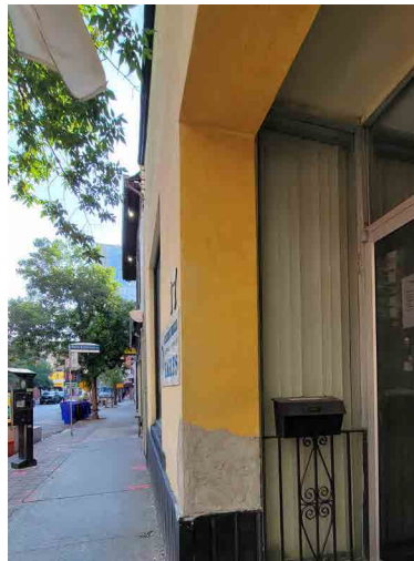
Figure 65: Stucco and cement repair (ERA, 2022).
