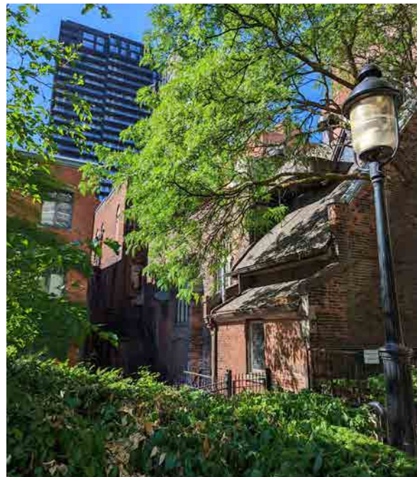
Figure 32: Partial east elevation (ERA, 2022).
