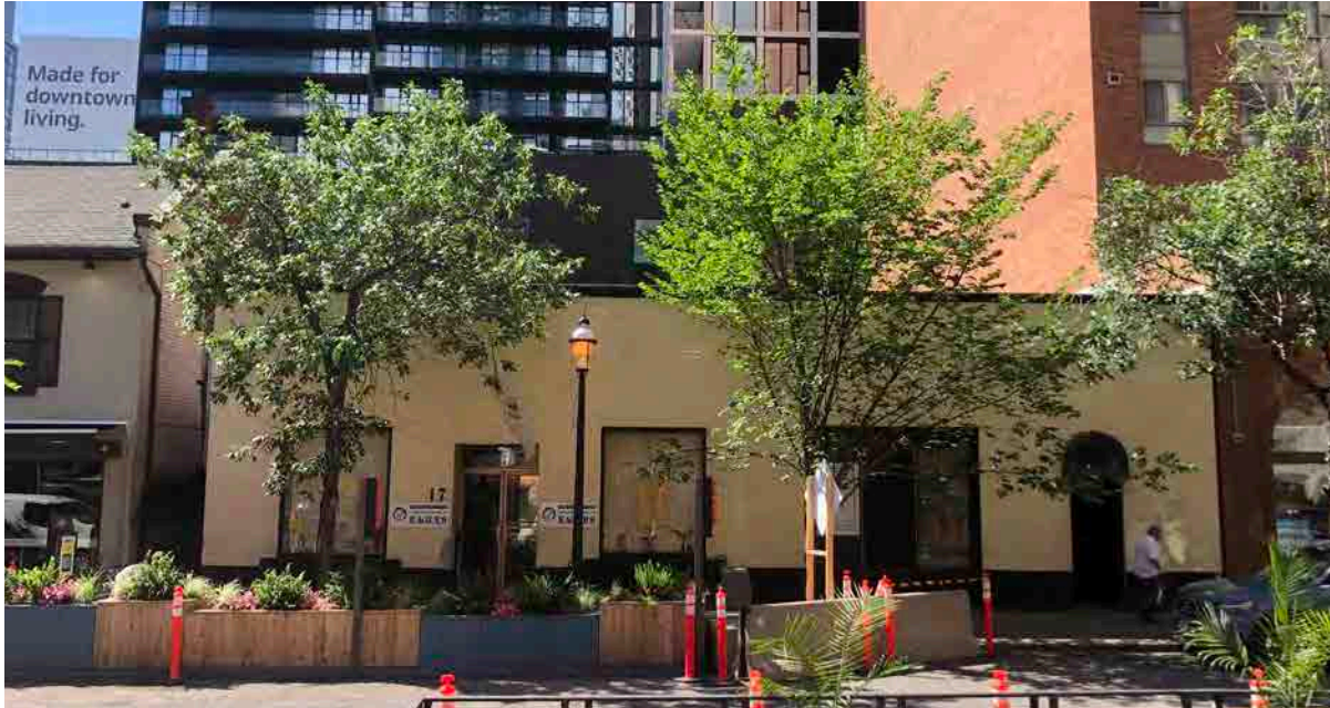
Figure 21: North elevation (ERA, 2022).
