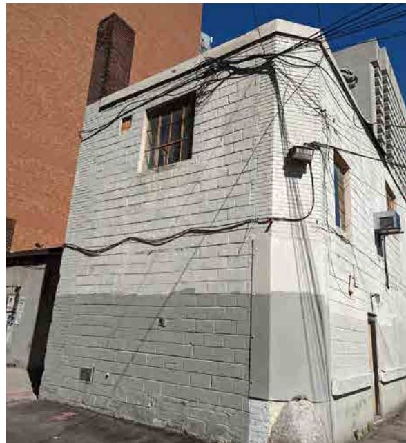
Figure 20: South elevation (ERA, 2022).
