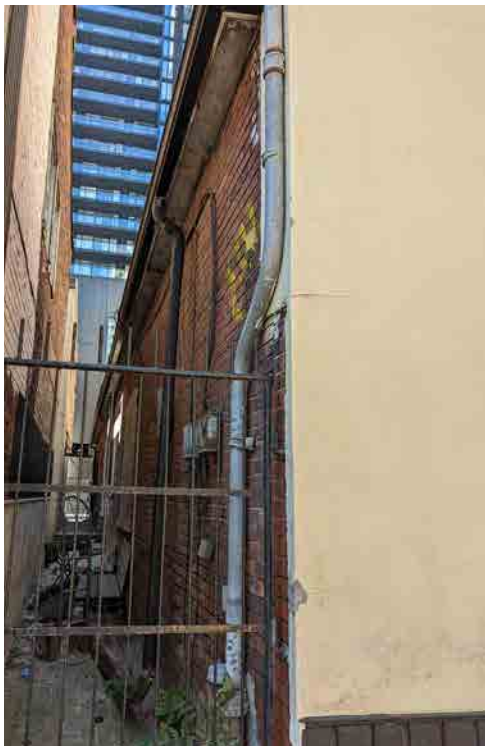
Figure 22: Partial east elevation (ERA, 2022).
