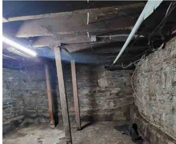
Figure 59: Wood posts shoring up sagging floor (ERA, 2022).
