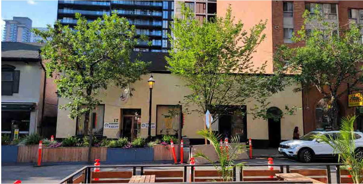
Figure 62: North elevation (ERA, 2022).
