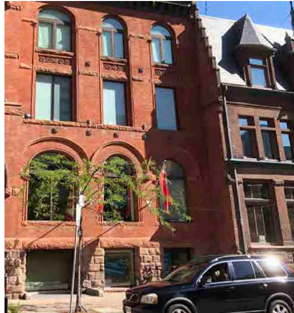
Figure 30: Partial west elevation (ERA, 2022).
