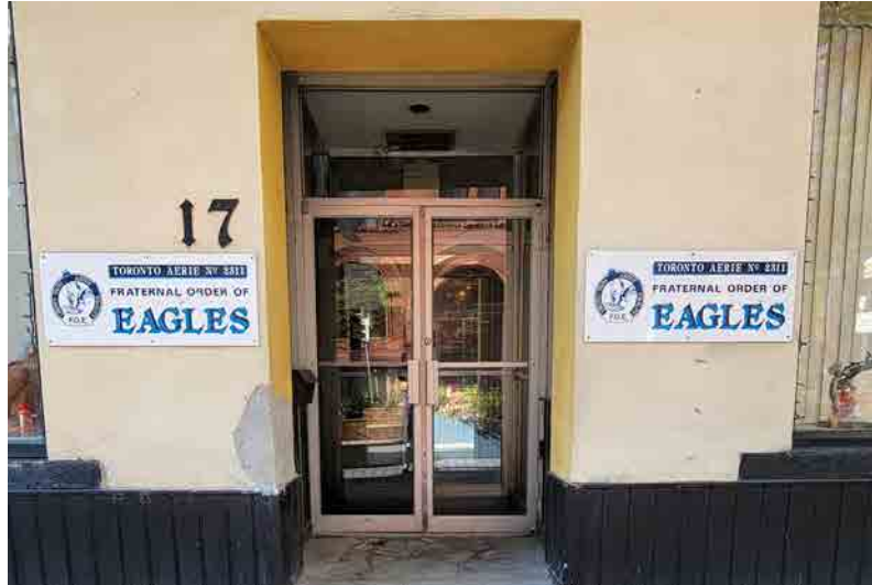
Figure 63: Aluminium doors and vestibule with glazing in fair condition. Cement stucco repairs visible. Stone step is in poor condition (ERA, 2022).
