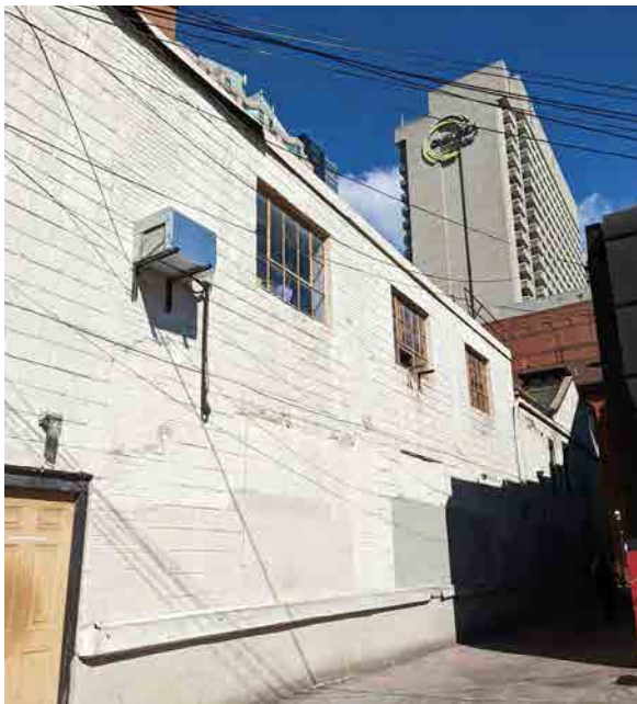
Figure 19: Partial east elevation (ERA, 2022).
