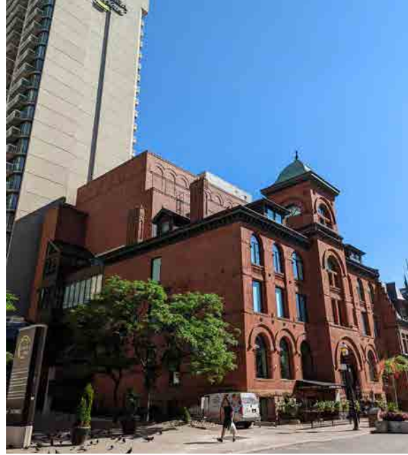
Figure 34: South and partial west elevation of 18 Elm Street (ERA, 2022).
