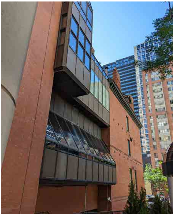
Figure 35: West elevation (ERA, 2022).
