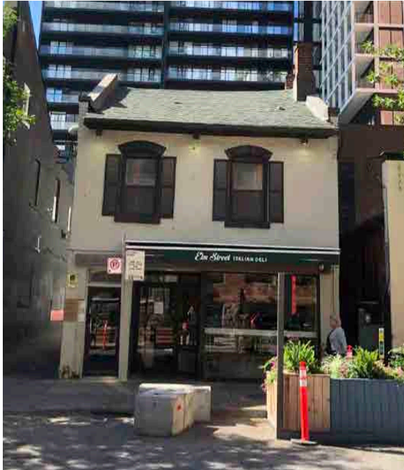
Figure 17: North elevation (ERA, 2022).
