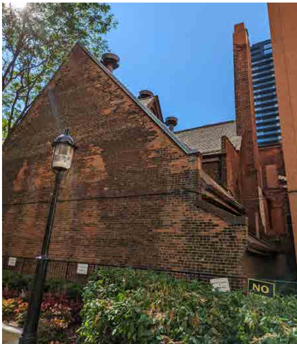
Figure 31: North and partial west elevation (ERA, 2022).
