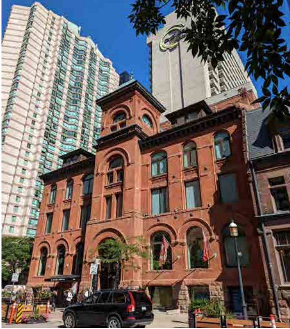
Figure 33: South elevation (ERA, 2022).
