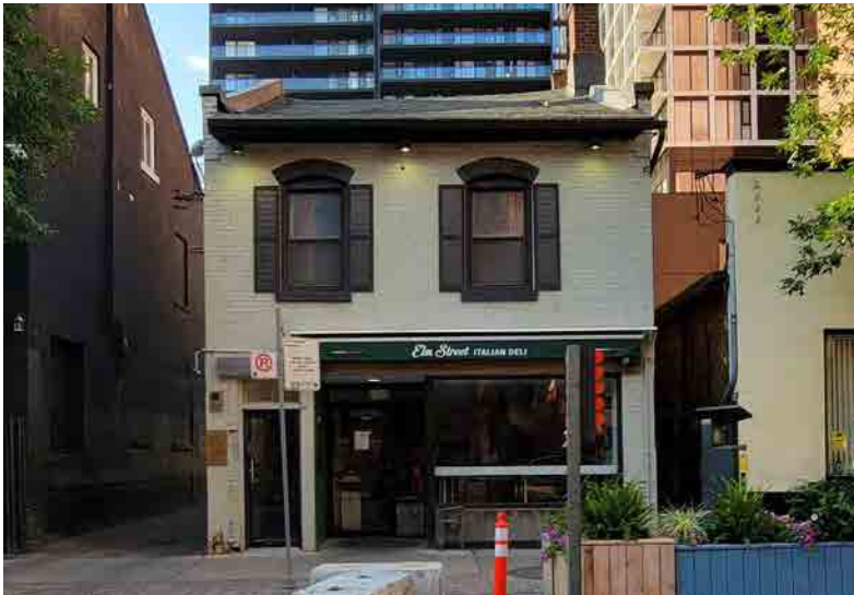
Figure 42: North elevation (ERA, 2022).
