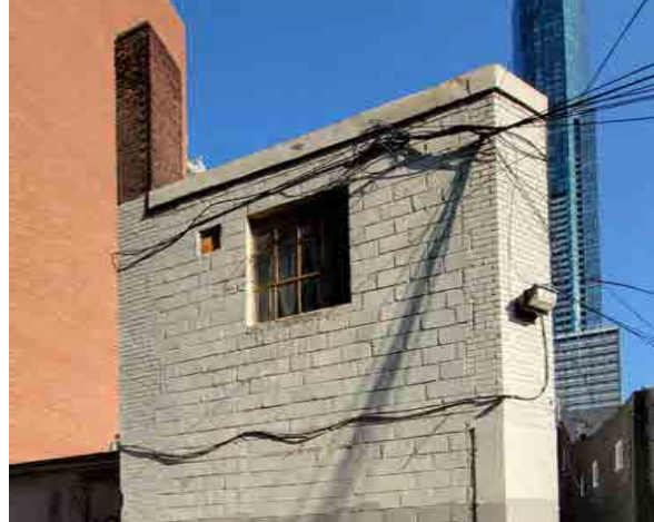
Figure 58: Parapet wall with metal flashing (ERA, 2022).
