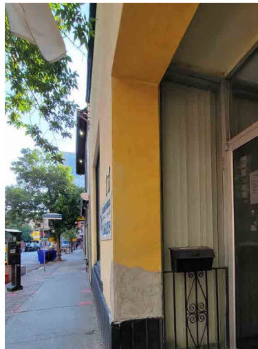
Figure 65: Stucco and cement repair (ERA, 2022).
