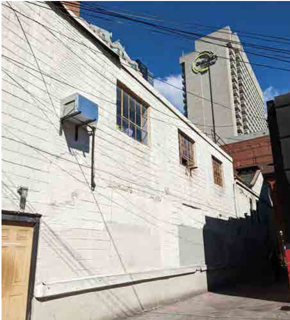
Figure 9: Partial east elevation (ERA, 2022).
