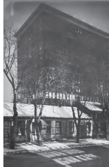
Figure 22: T Eaton's Co. factory as seen from Terauley Street in 1930 (City of Toronto Archives).
