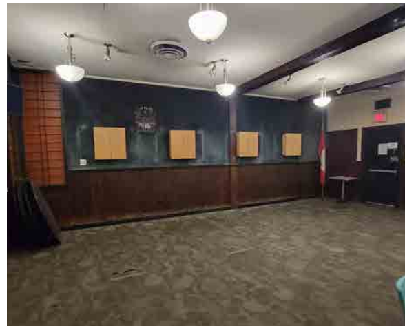
Figure 76: Materials are mixed and dated with dropped ceiling and carpet floor (ERA, 2022).
