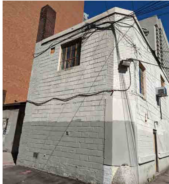
Figure 10: South elevation (ERA, 2022).
