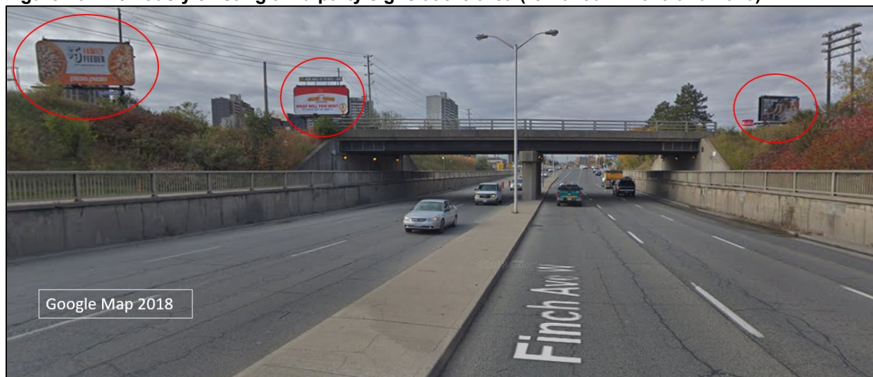
Figure 10- Previously existing third party signs at the area (removed in 2019 and 2020)
