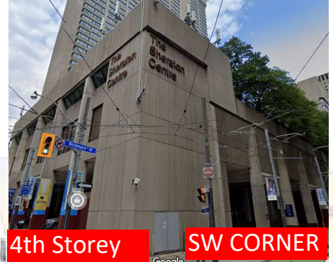
Sheraton on Richmond St W - 180 m away from N.B.
