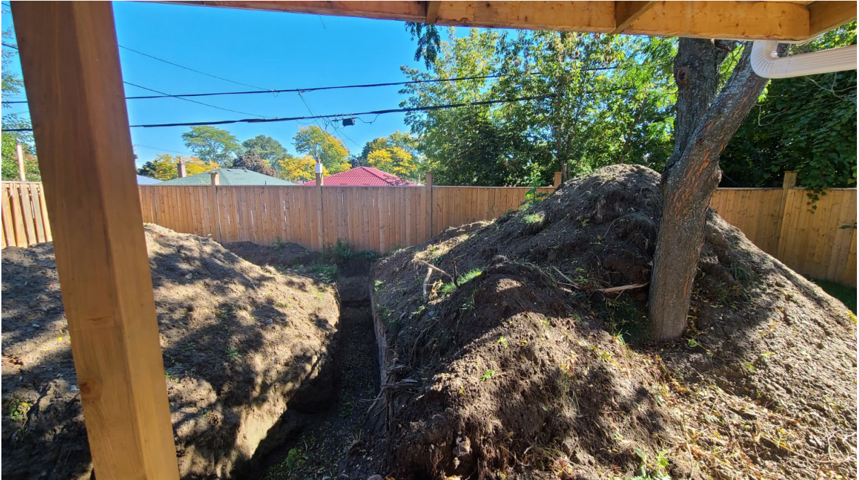
Attachment 5: Rear yard fence
