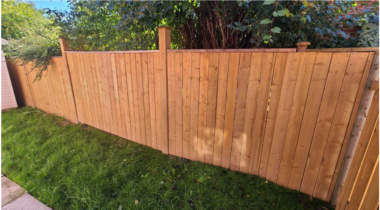
Attachment 3: Rear yard fence
