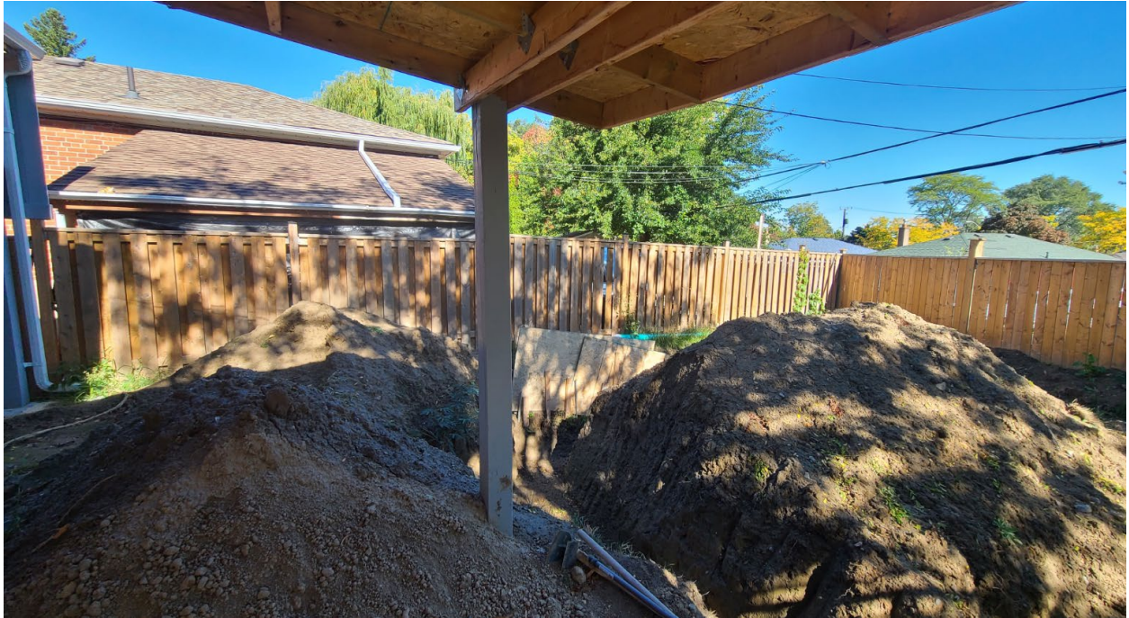
Attachment 4: Rear yard fence
