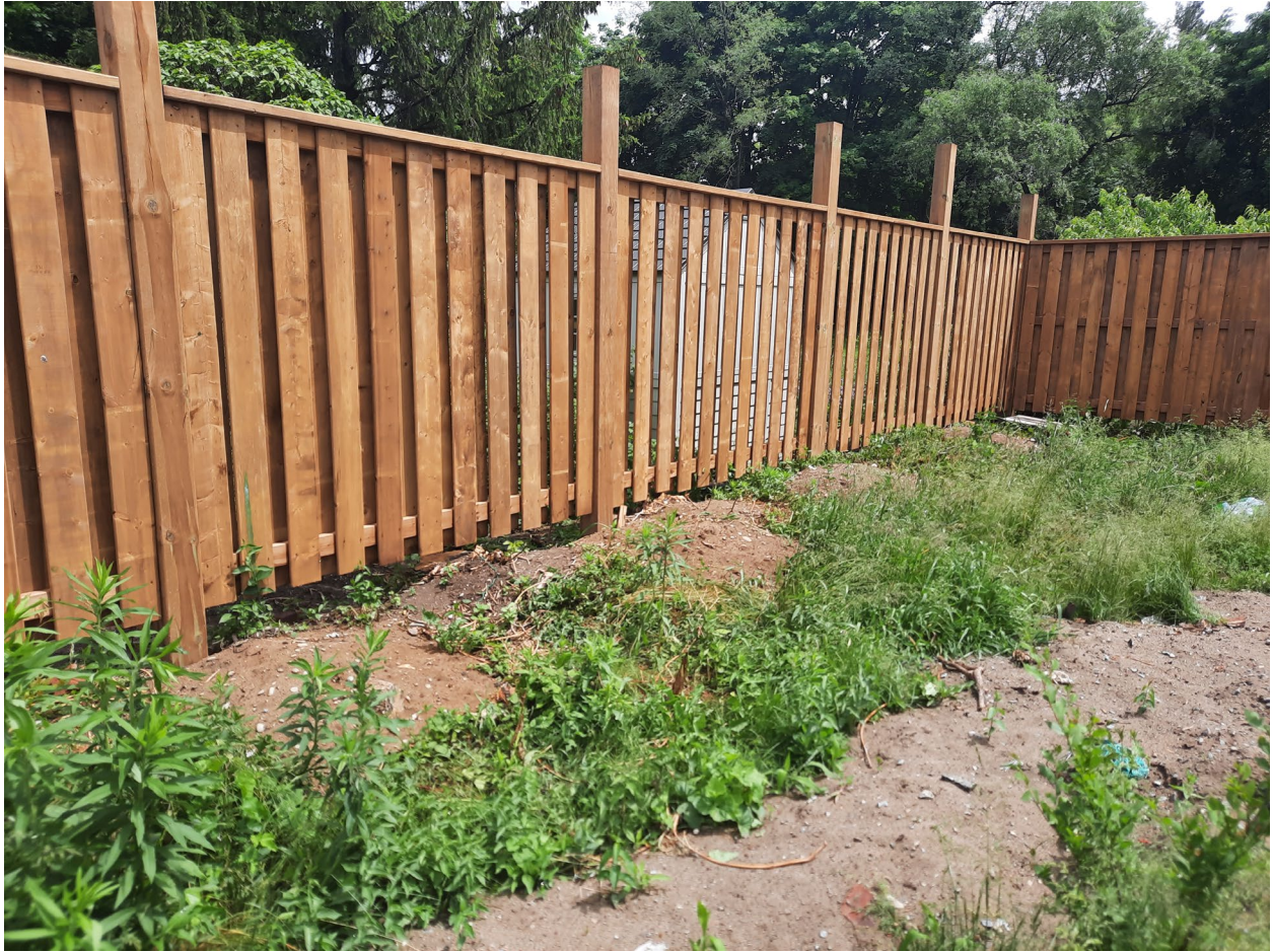
Attachment 8: Height of fence with posts and space between ground and fence
