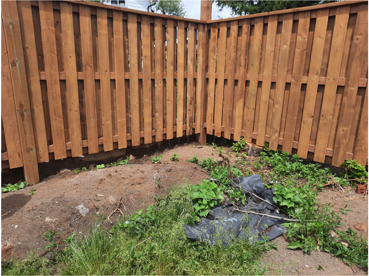
Attachment 6: Height of fence with posts and space between ground and fence
