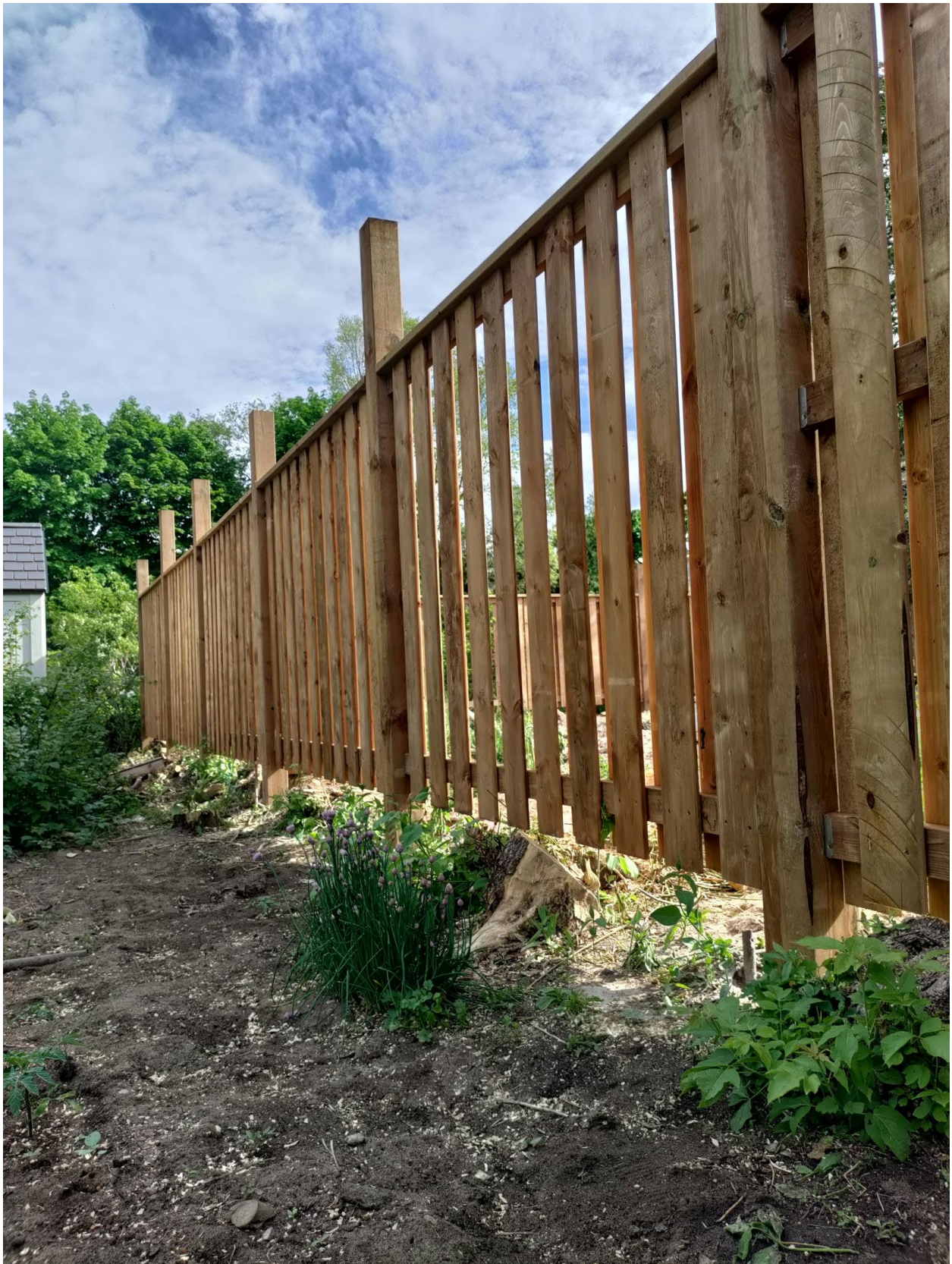
Attachment 5: Height of fence with posts and space between ground and fence
