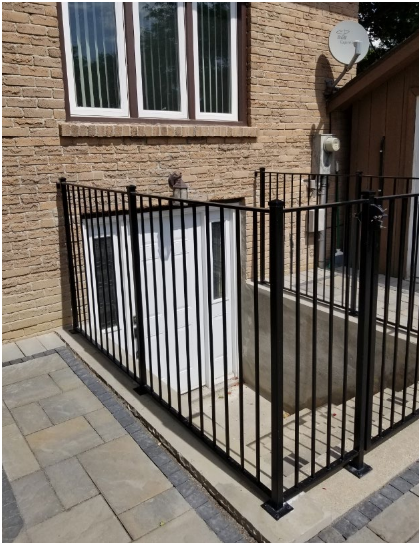
Attachment 4: Rear of house – basement egress south side
