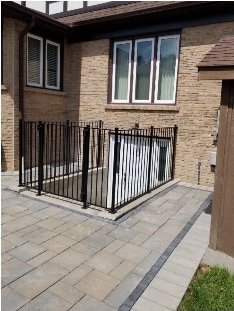
Attachment 3: Rear of house – basement egress south side
