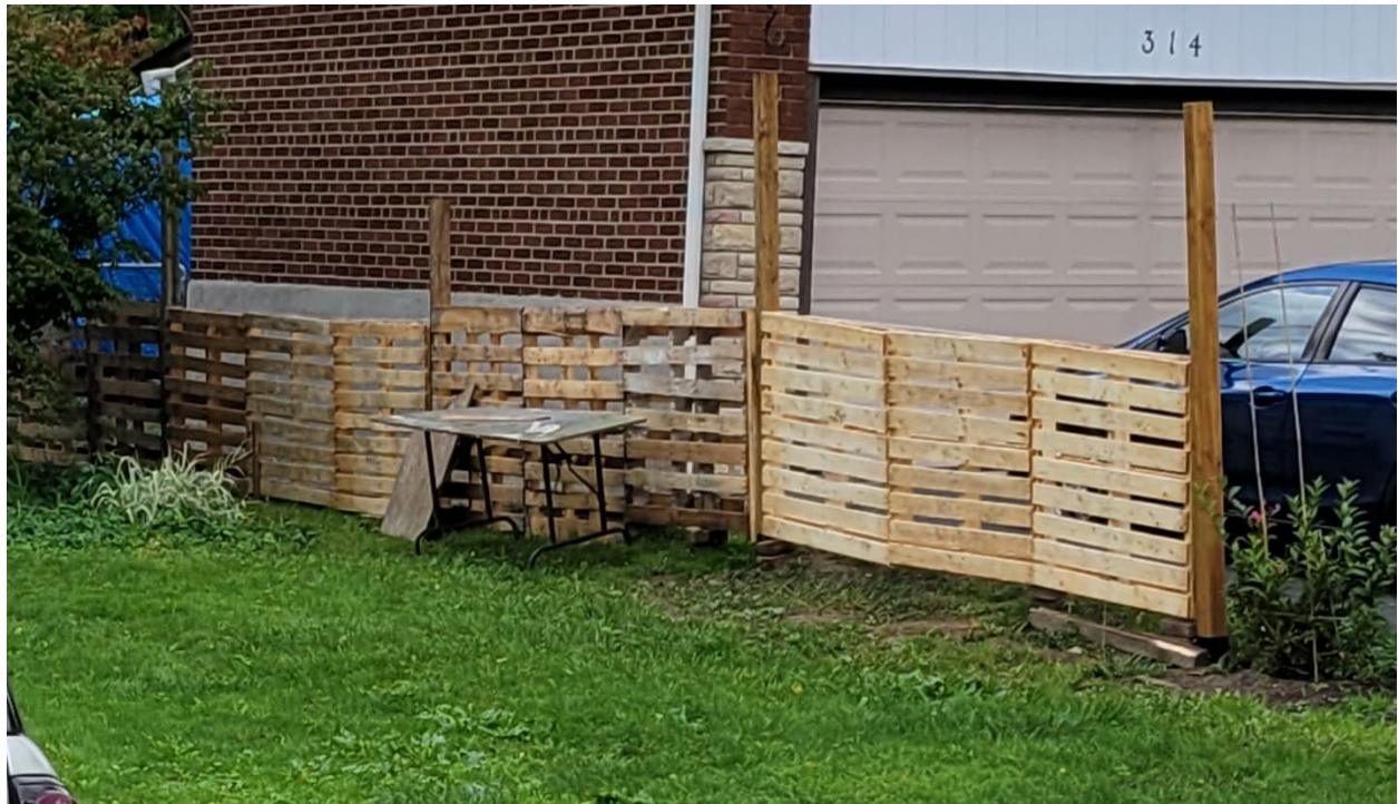
Attachment 2: Photo of fence – 312 Morrish Road (Taken by MLS Officer Mike Worth at Time of Inspection) Front Fence (09/2022)
