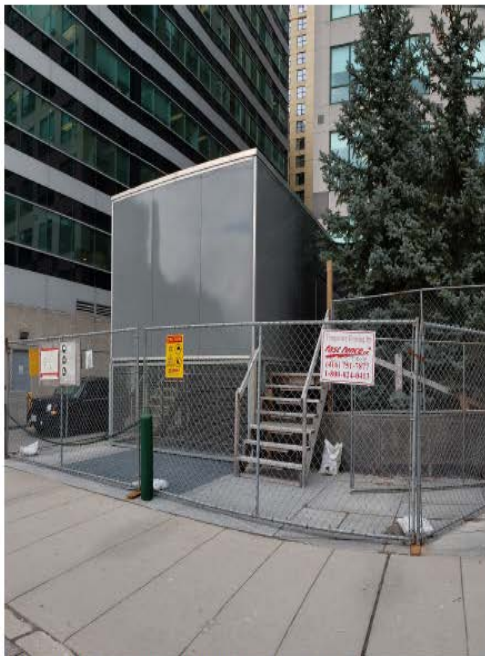
Existing Site Conditions showing temporary fencing.
