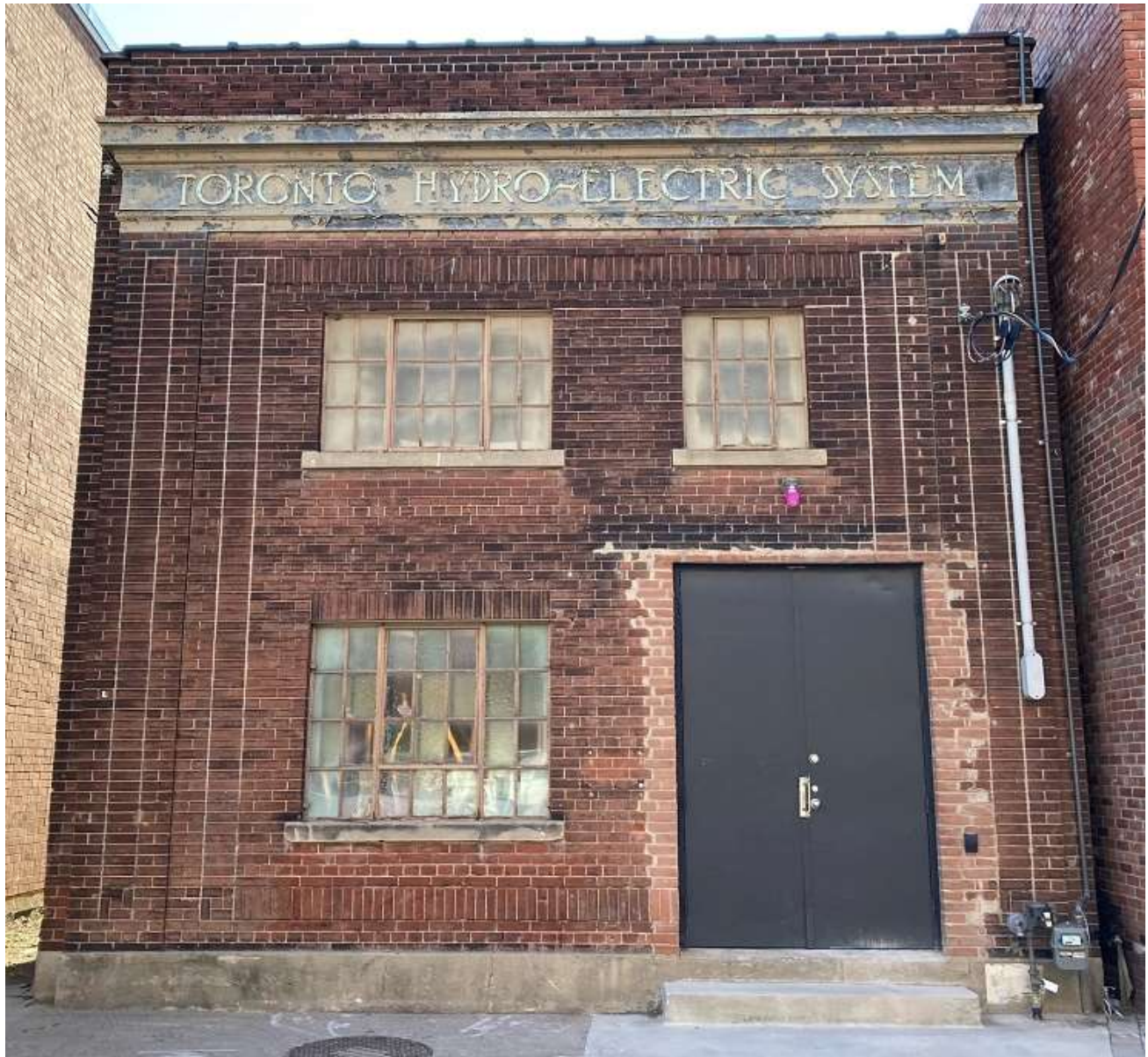
Photograph of the front/Portland Street of 18 Portland Street.
