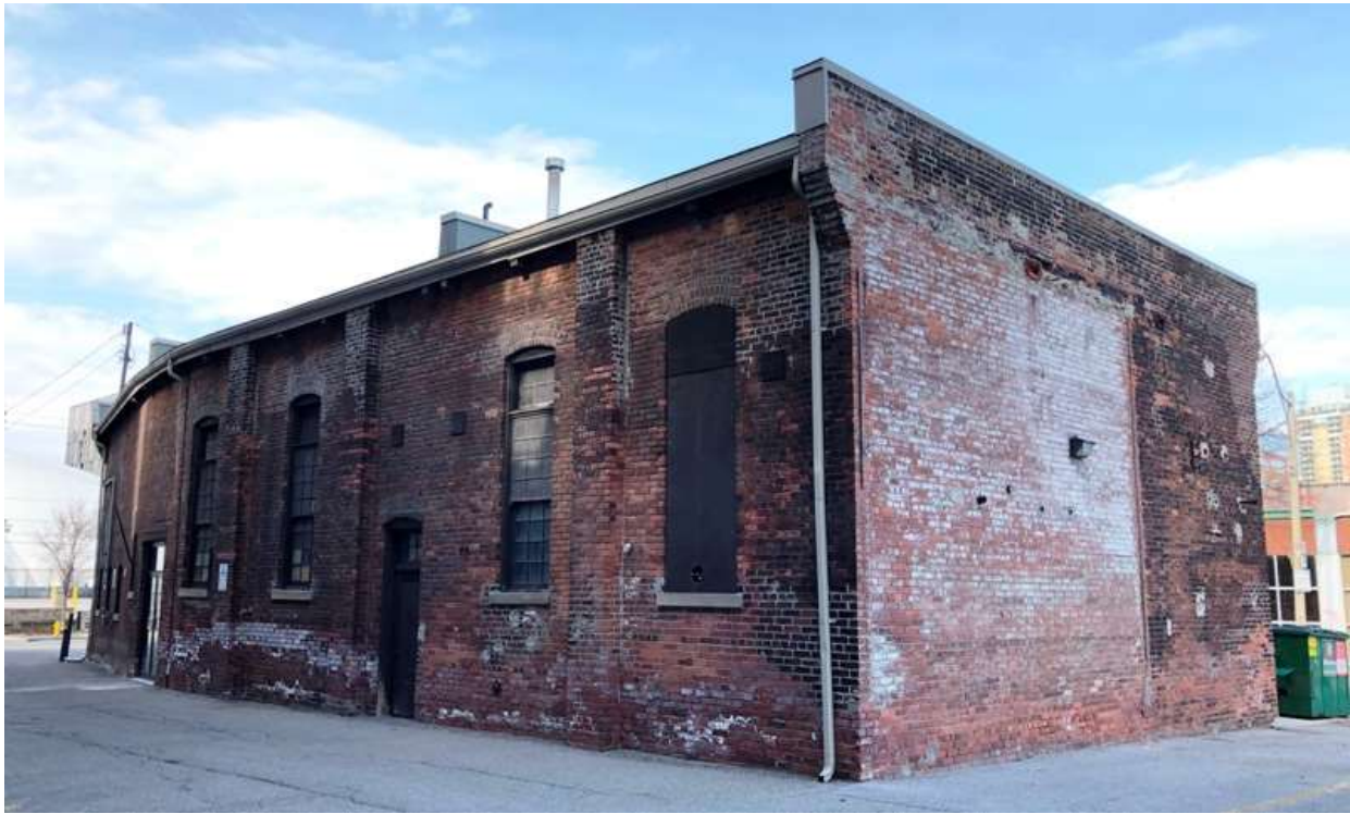
South-west facade of the powerhouse building (HP, 2020)
