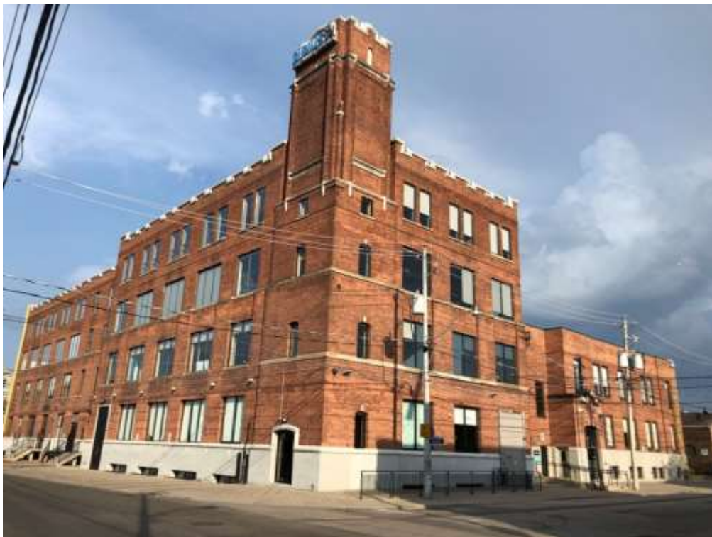
North and west facades at the intersection of Fraser Avenue and Liberty Street (HP, 2020)
