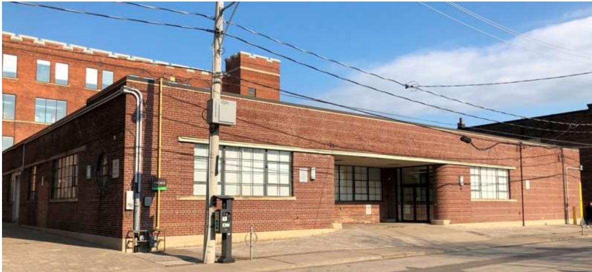
West and north facades of 41 Fraser Avenue (HP, 2020)
