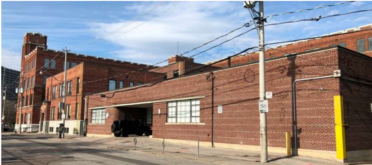
Looking north on Fraser with view of the 1941-2 Garage-Storage building at 41 Fraser with the office at 47 Fraser and the former factory at 135 Liberty Street (HP, 2020)
