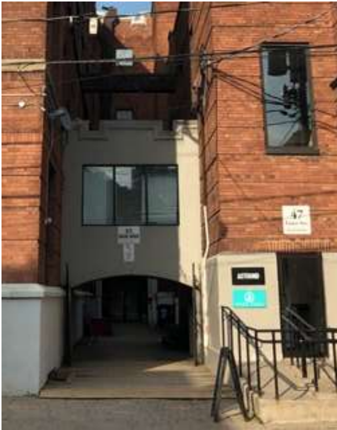
Bridge linking the former factory building at 135 Liberty Street with the former office building at 47 Fraser Avenue (HP, 2020)
