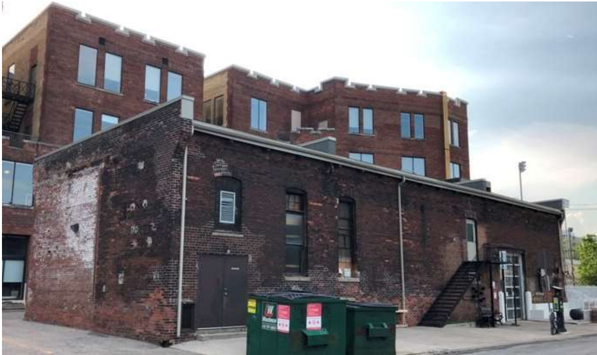
South and east facades of the powerhouse building (HP, 2020)
