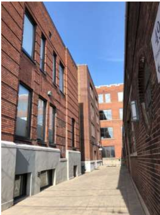
View (left) of the south facades of 47 and 49 Fraser Avenue along a passageway terminated by 53 Fraser Avenue. (HP, 2020)
