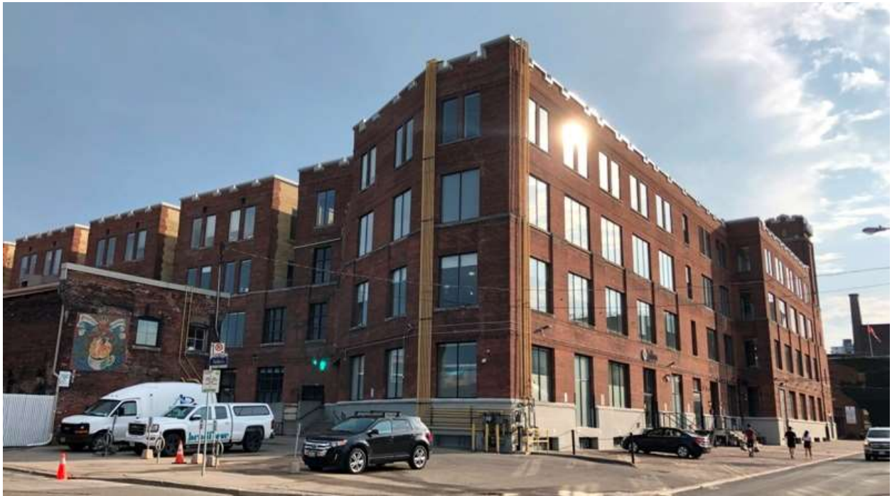
North-east corner of the factory at the intersection of Pardee Avenue and Liberty Street showing the angled end of the building with the powerhouse to the left (HP, 2020)
