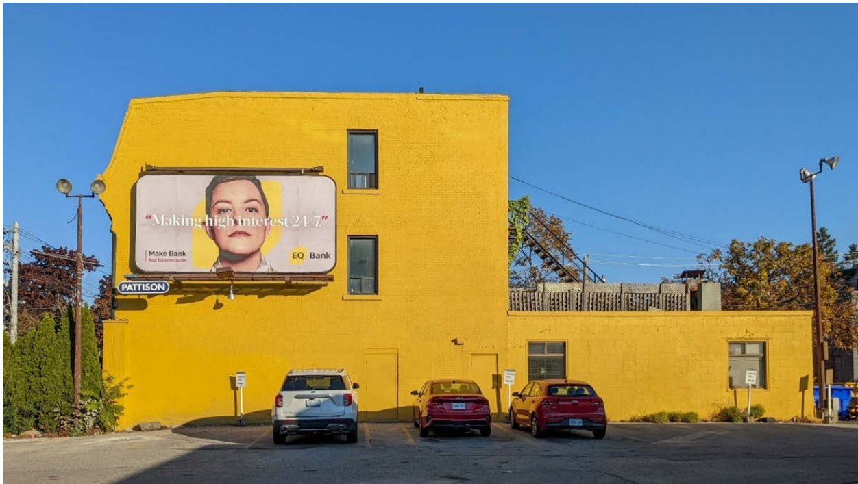
Side (south) elevation of 127 Strachan Avenue (Heritage Planning, 2022).
