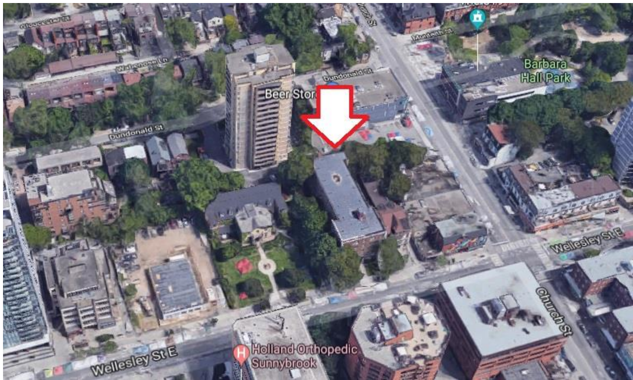
Aerial photograph showing the location of the heritage property at 64 Wellesley Street East (Google Maps).
