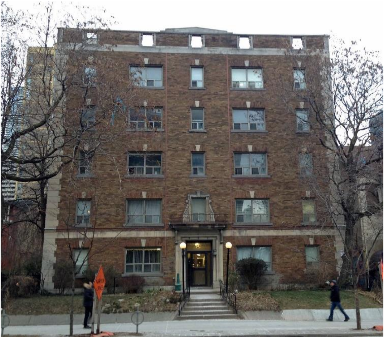
Photograph, front (south) elevation, 64 Wellesley Street East (Heritage Planning, 2019)
