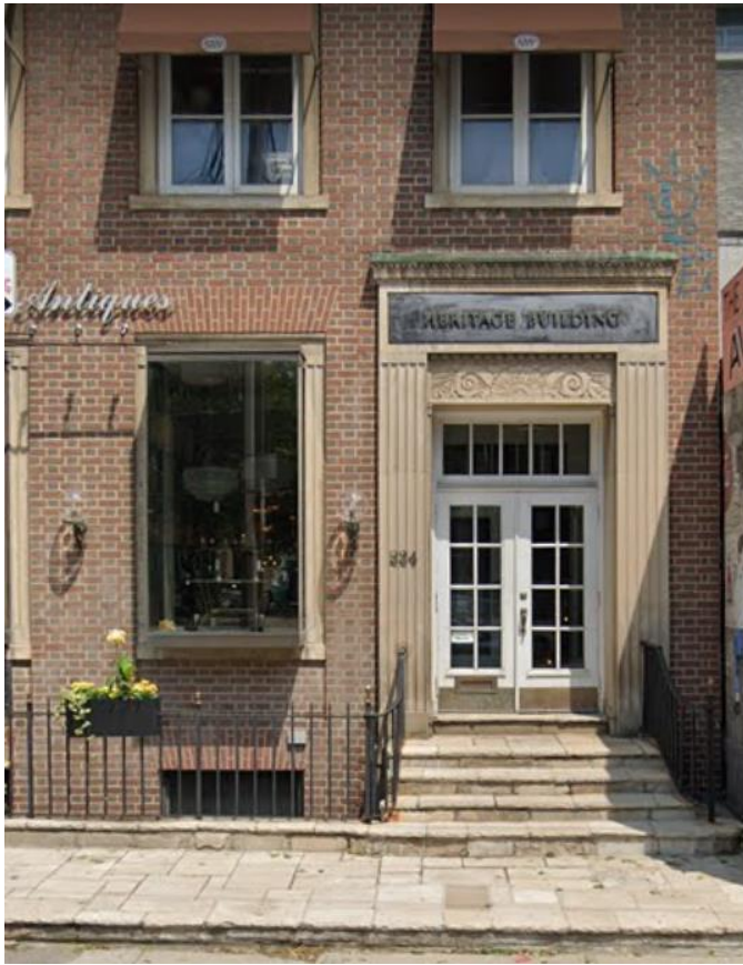
224 Davenport Road: detail of raised main entrance on the principal (south) elevation showing the stone door surround with fluting pilaster and carved inset, decorative window surrounds and metal railing. (Heritage Planning, 2021)
