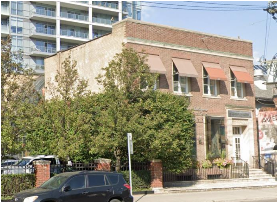
Current image of the Canada Bread Building at 224 Davenport Road showing the stone and copper cornice line on the principal (south) elevation and buff brick cladding on the west elevation. (Heritage Planning, 2021)
