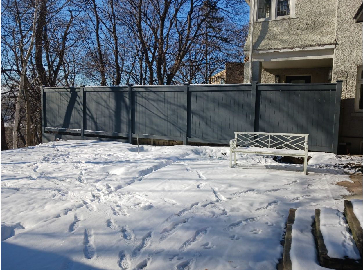
Photograph of Existing Fence
