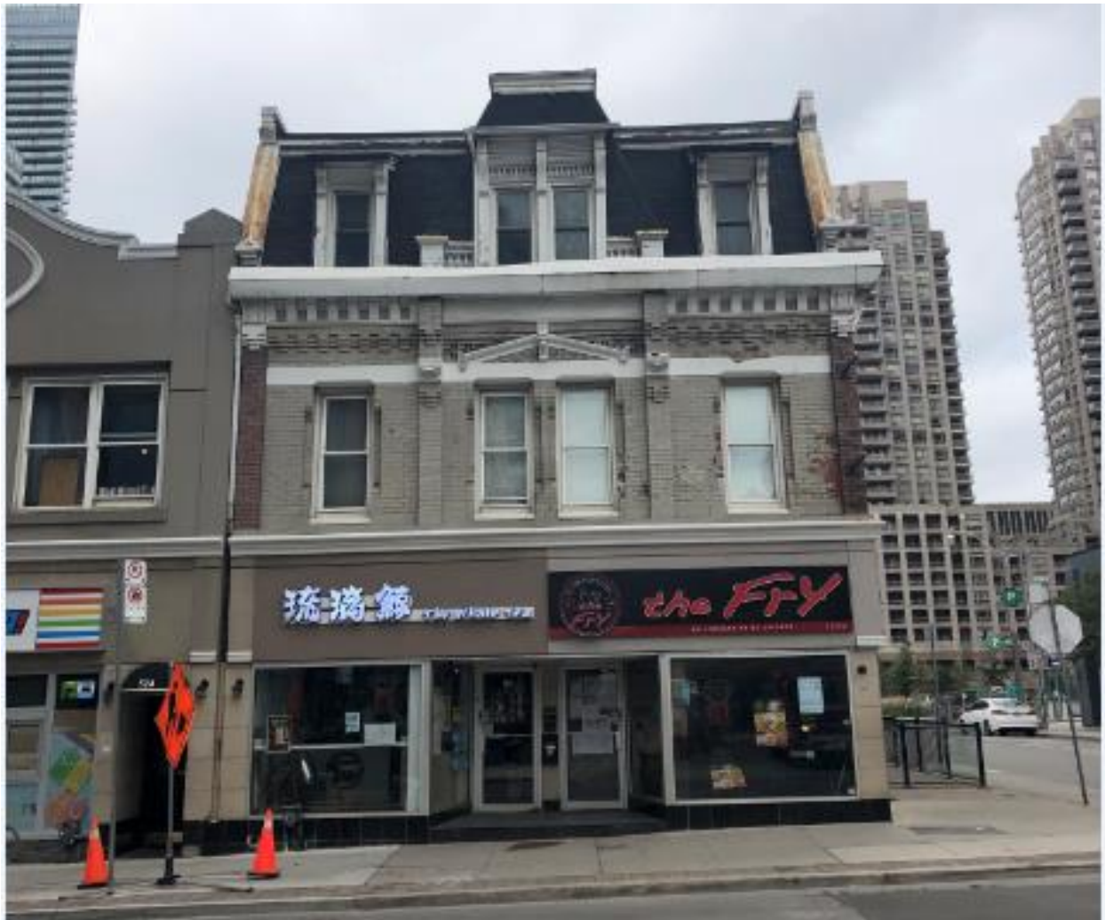
Figure 5. Principal (east) elevation of 526-528 Yonge Street looking west (Heritage Planning, 2021).
