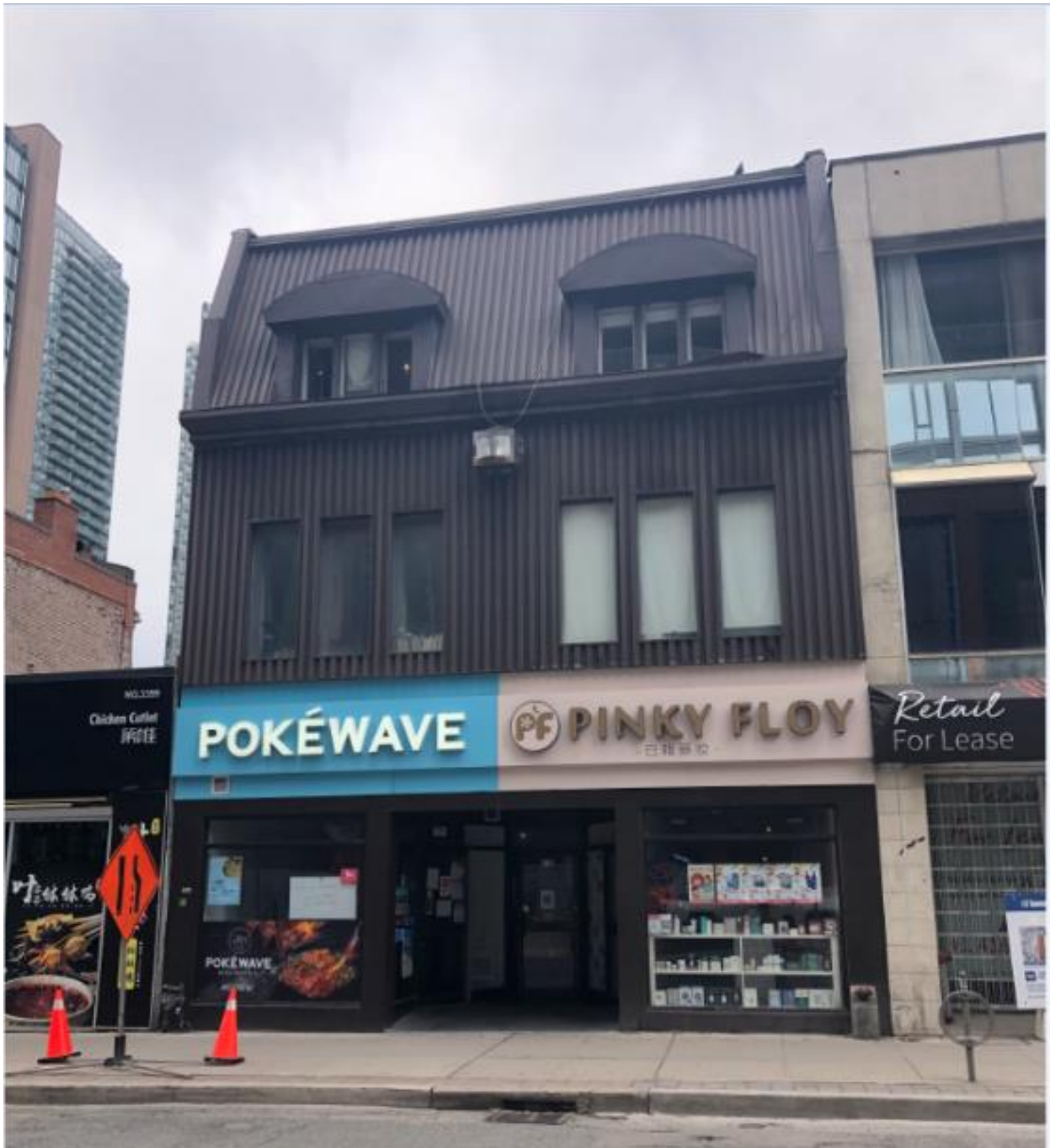
Figure 4. Principal (east) elevation of 514-516 Yonge Street looking west (Heritage Planning, 2021).
