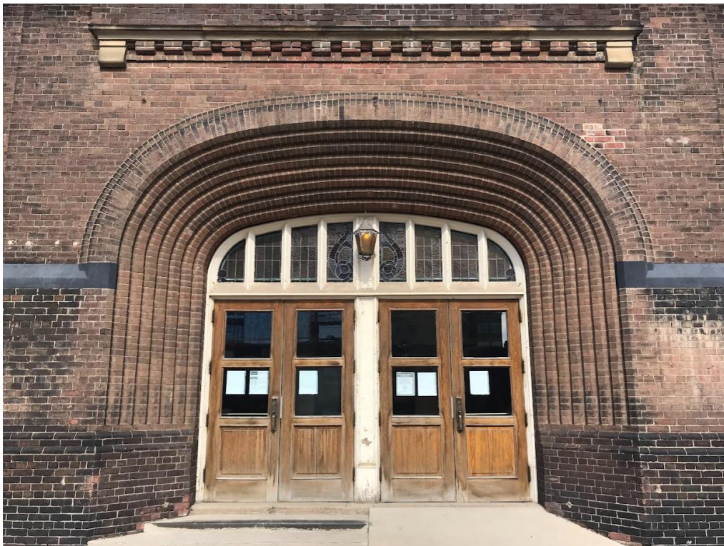
The main entrance on the principal (west) elevation (Heritage Planning, 2022)
