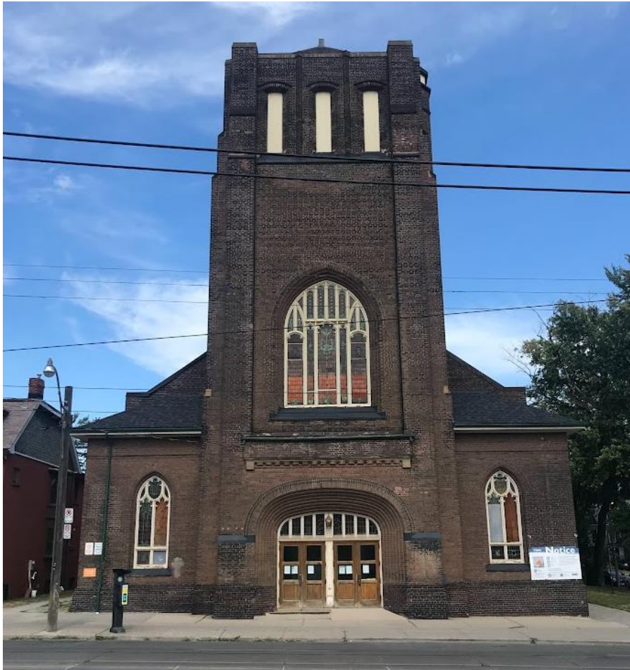
Principal (west) elevation of the church with its centred tower and flanking transepts (Heritage Planning, 2022)
