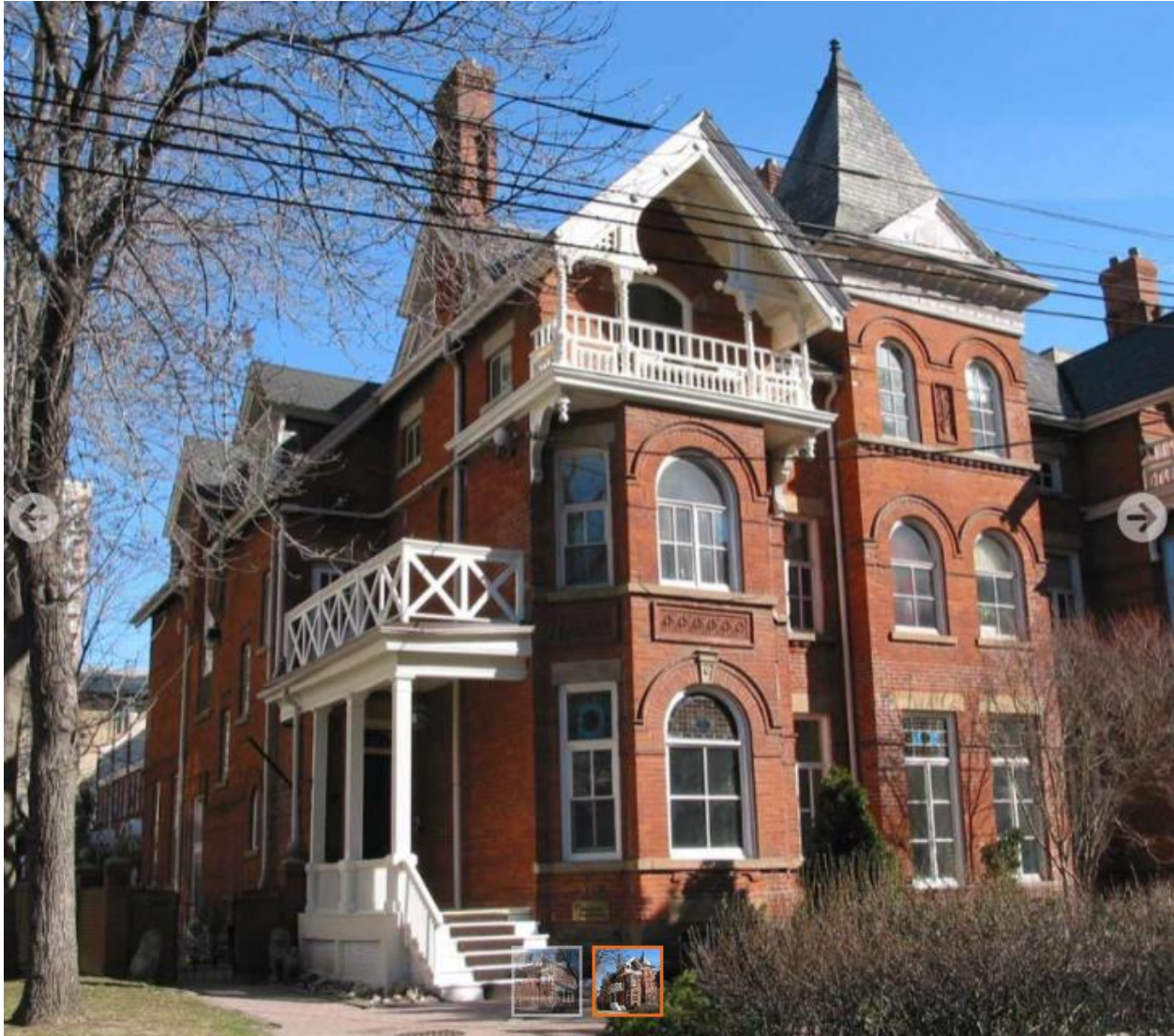
90A Isabella Street (left) Source: Bob Krawczyk/Architectural Conservancy of Ontario
