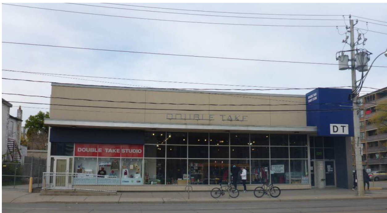
Existing building at 310 Gerrard Street East. (Design Workshop Architects, 2021)
