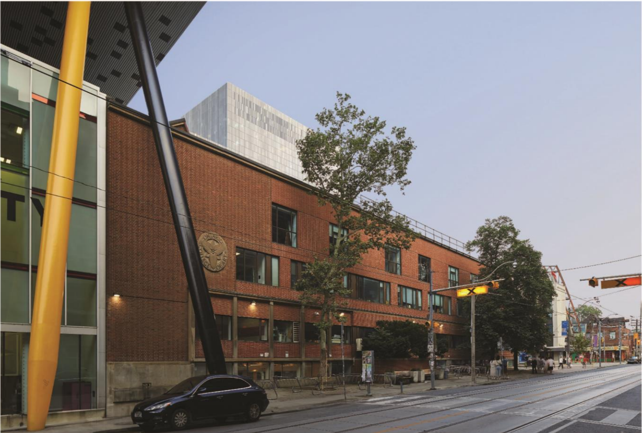
Attachment 10: Rendering of Proposal in Context (view from McCaul Street looking Northwest)
