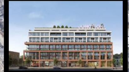
7. 2720-2730 Dundas St W 9-storays (Under Construction)
