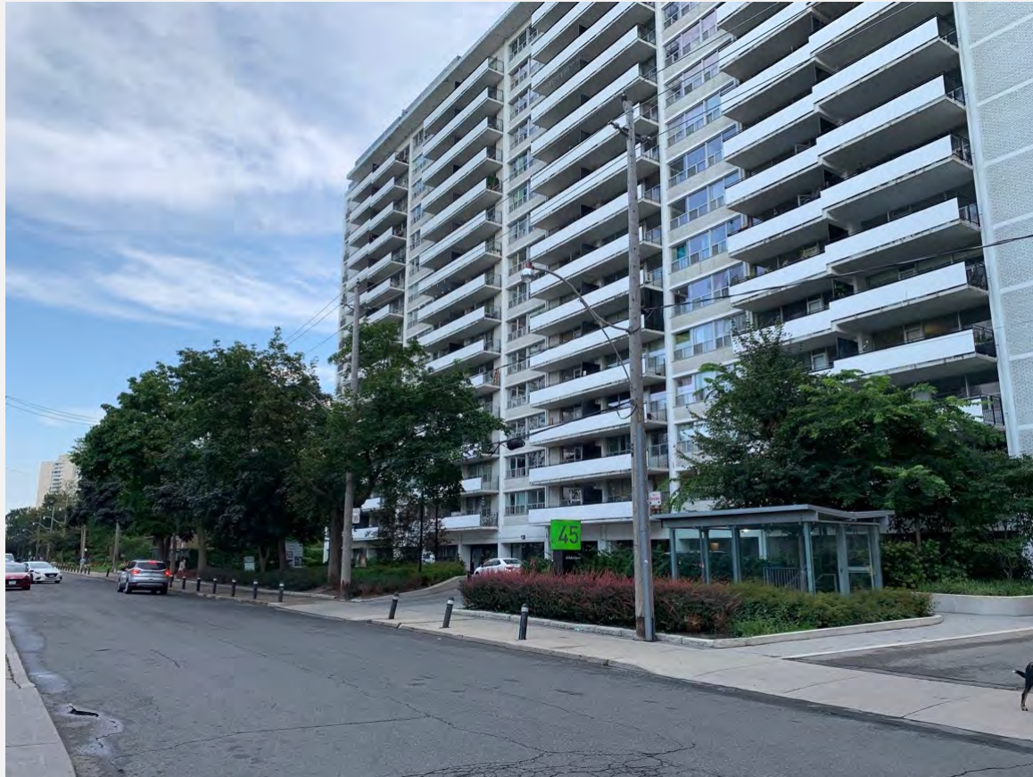
45 Balliol Street – Apartment Block
