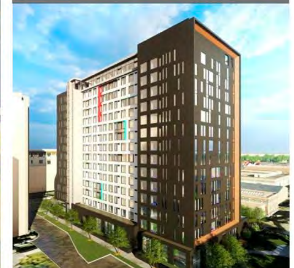
Birchmount Green, Toronto • 220 Affordable Units • Under Construction
