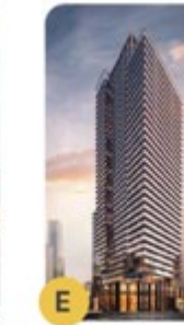
E Halo Residences on Yonge -480- 494 Yonge Street and 3 Grosvenor Street 38 Storeys Under Construction
