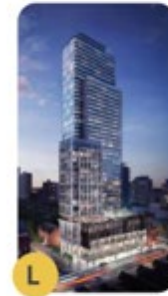
L The Clover on Yonge - 587-599 Yonge Street, 2-4 Dundas Street, and 7-9 Gloucester Street 44 Storeys Under Construction
