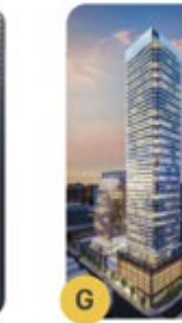
G TeaHouse - 501- 521 Yonge Street, 6-8 Alexander Street, and 23 Maitland Street 25 and 52 Storeys Built
