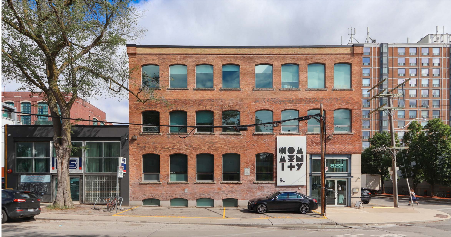
View looking north of 822 and 828 Richmond Street West
