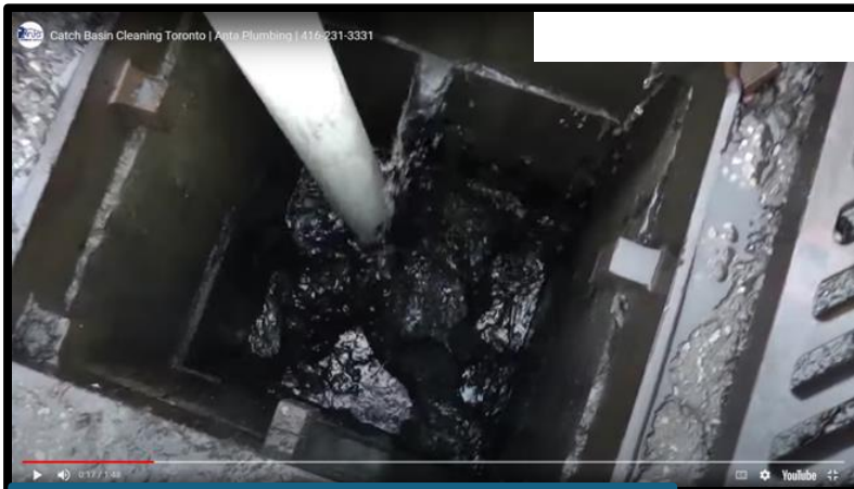
Woo-hoo!! Modern technology. Catch basin suction cleanout by vacuum truck. Far easier than the long-handled shovels used in the 1950s.
