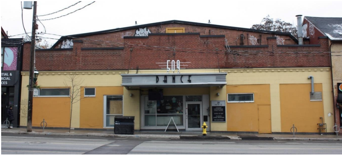
Main (west) façade, 2023 (Heritage Planning)
