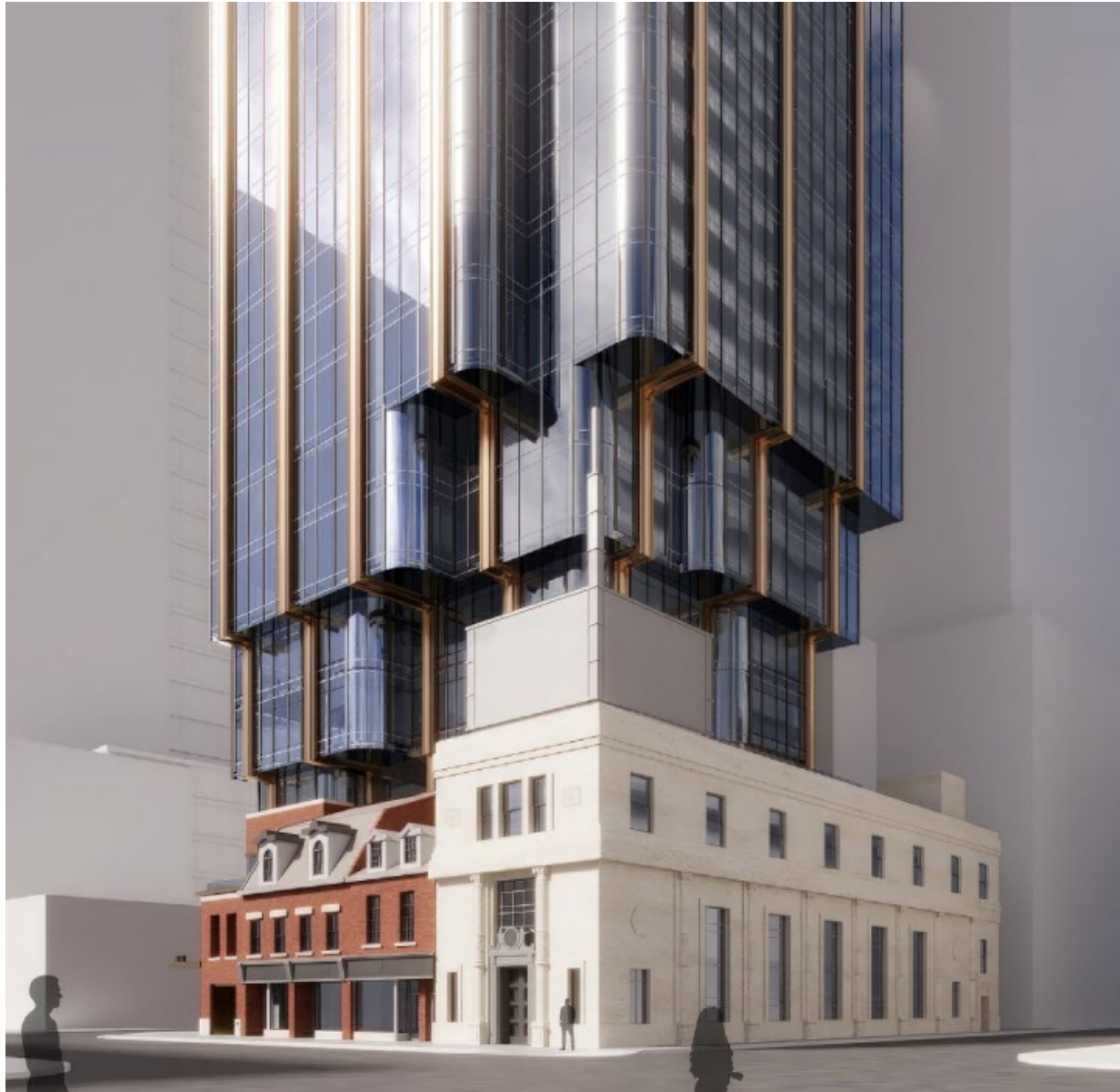
Render looking southwest towards corner property at 378 Yonge Street. Note proposed Cantilevers over Yonge Street frontage. (Dialog Architects)
