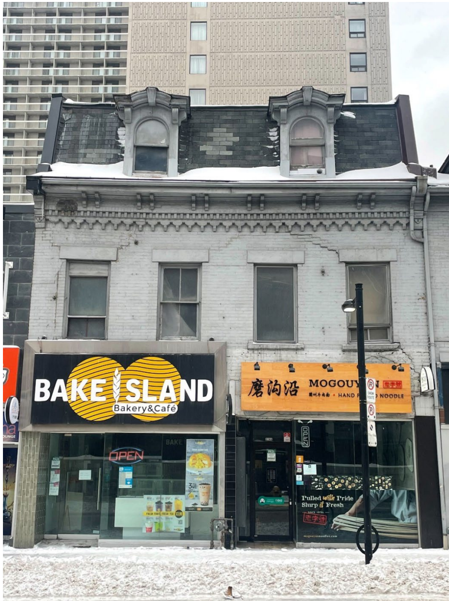
Photo of 374 Yonge Street, looking at east/front façade on Yonge Street (Heritage Planning)
