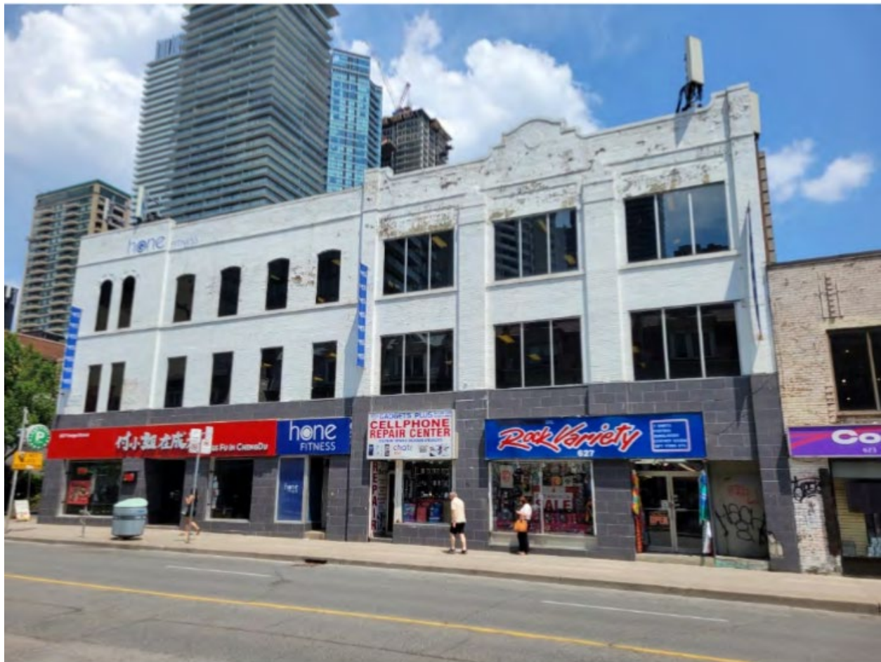
Principal (West) Elevation of 625 Yonge Street (Source: HIA prepared by VG Architects Ltd.,).
