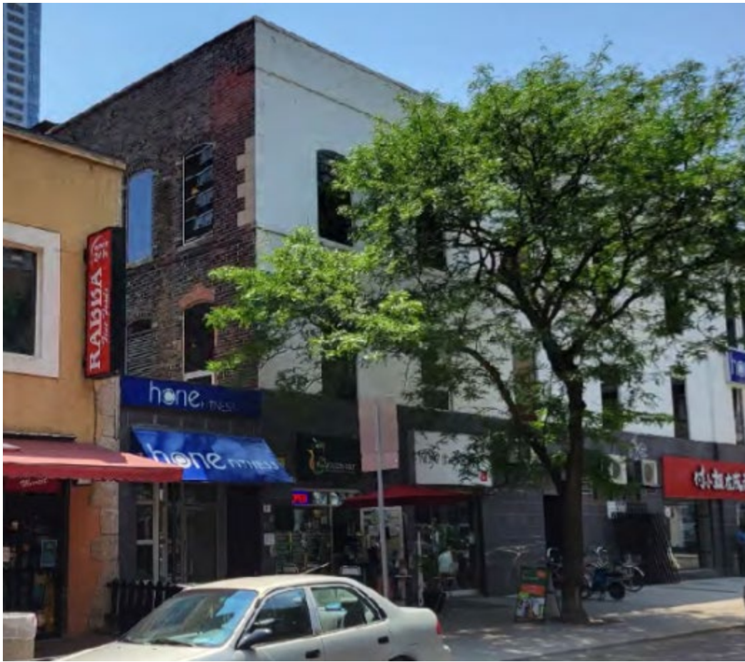
North and East Elevations of 625 Yonge Street (Source: HIA prepared by VG Architects Ltd.,).
