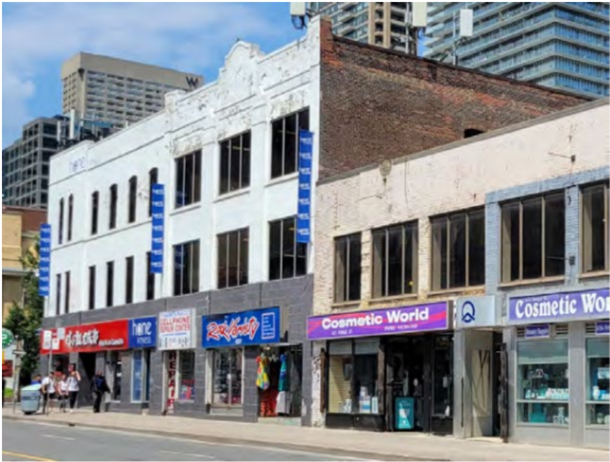
Principal (West) and South Elevations of 625 Yonge Street (Source: HIA prepared by VG Architects Ltd., 2023).
